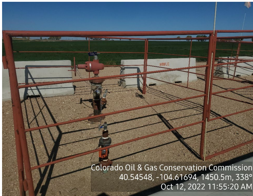
Photo 1: TA Wellhead, NO SIGNAGE
