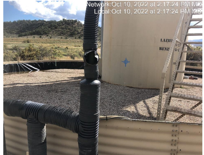
Photo #8019 Heating insulation open ended and not capped.
