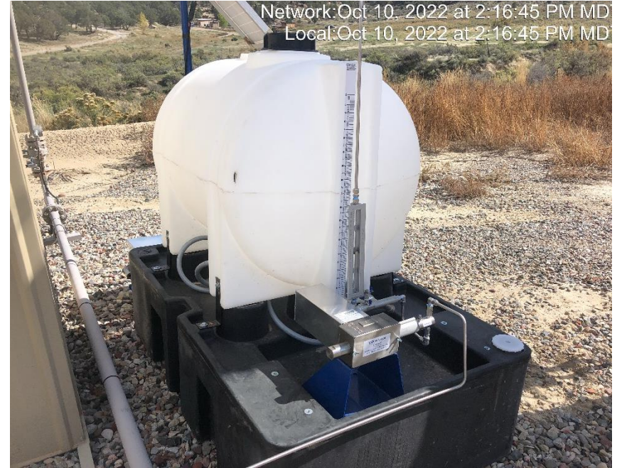
Photo #8017 Chemical tank missing required information.
