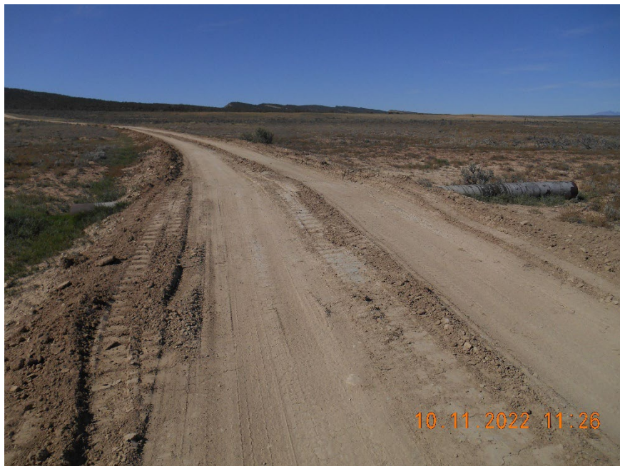
Culvert on access road.
