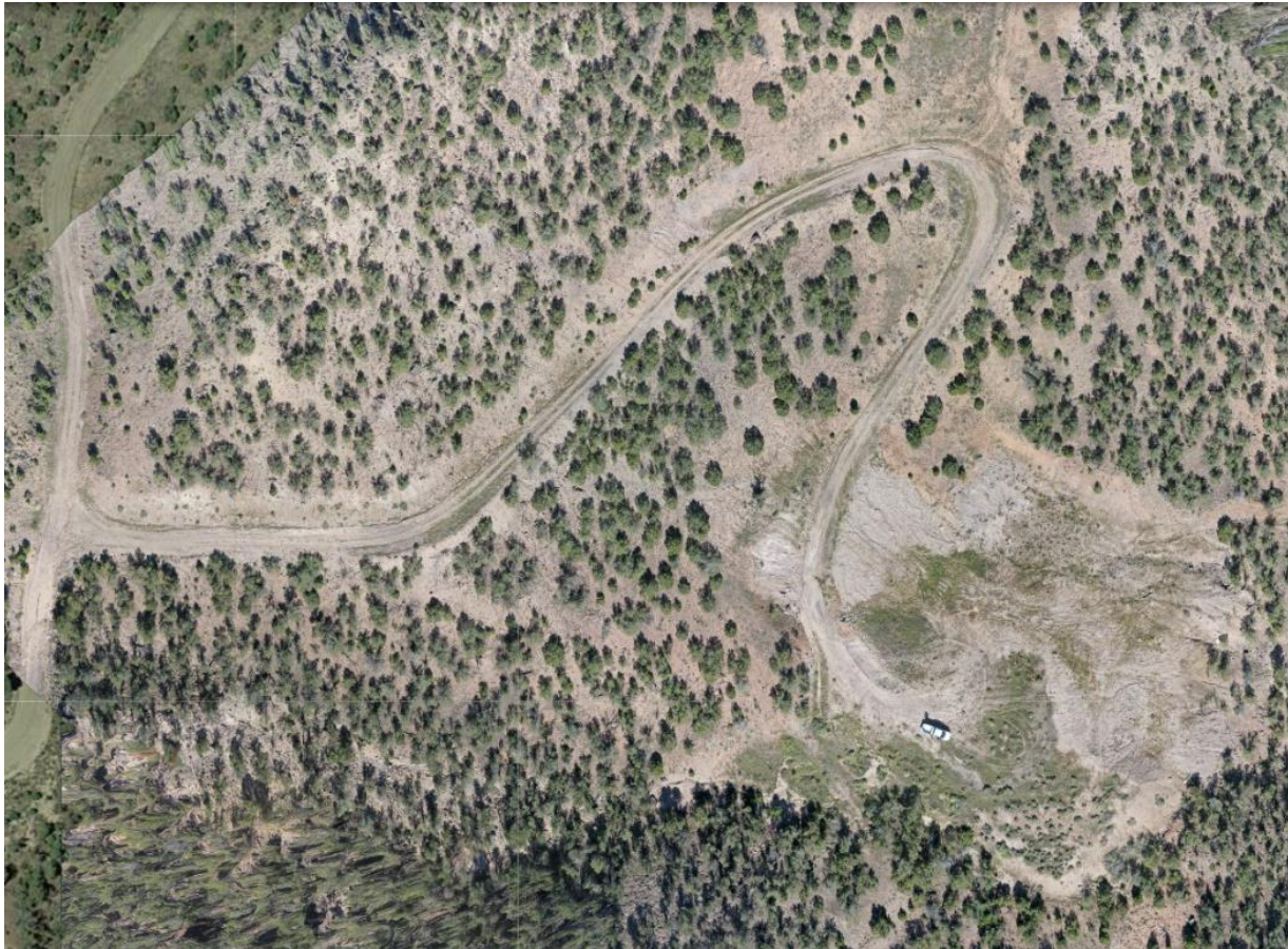
Photo 1: Aerial imagery of Location dated 10/11/2022 taken with use of a sUAS. Image shows overview of the Location and access road; final reclamation has not been conducted in accordance with 1004 requirements.
