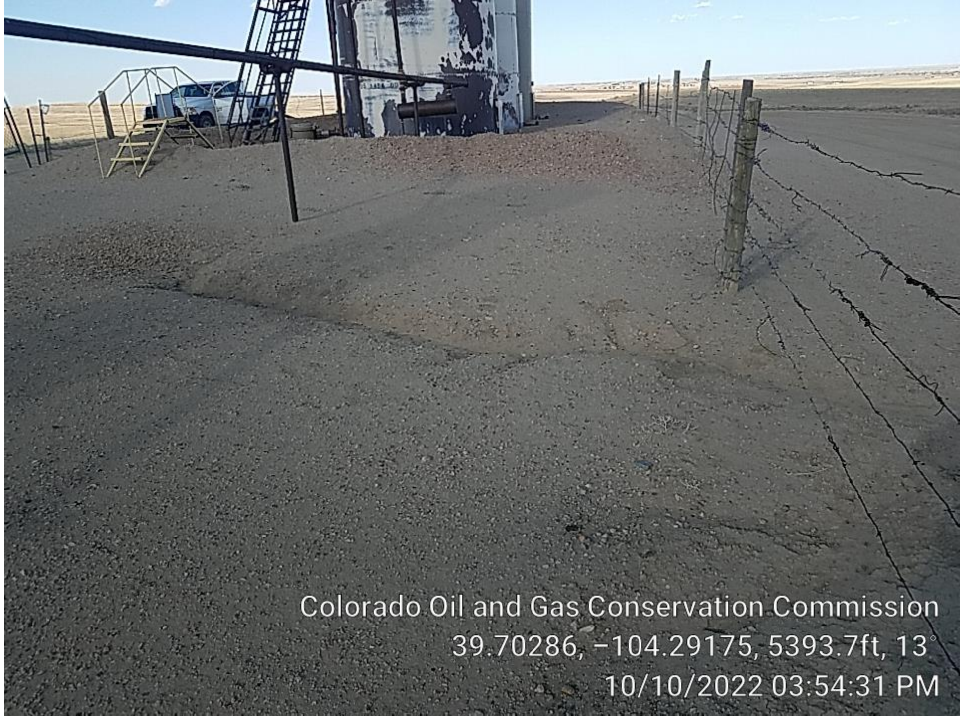
Erosion rill and sediment transport at tank battery.
