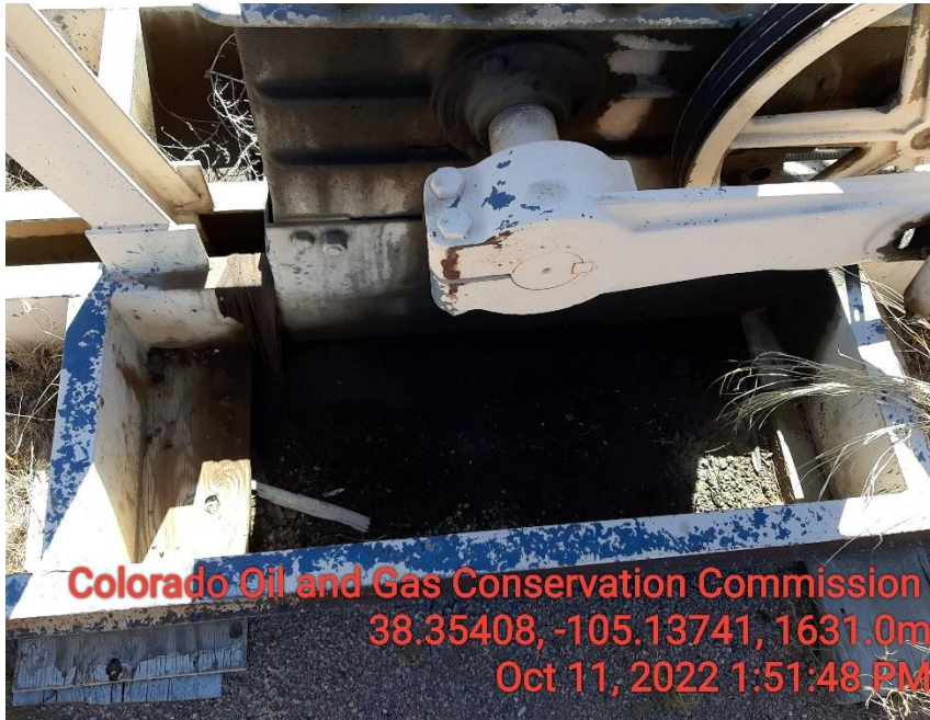
Photo 3 stained soil around PU
