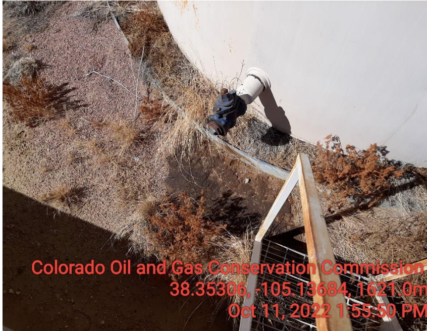
Photo 7 stained soil crude oil load line
