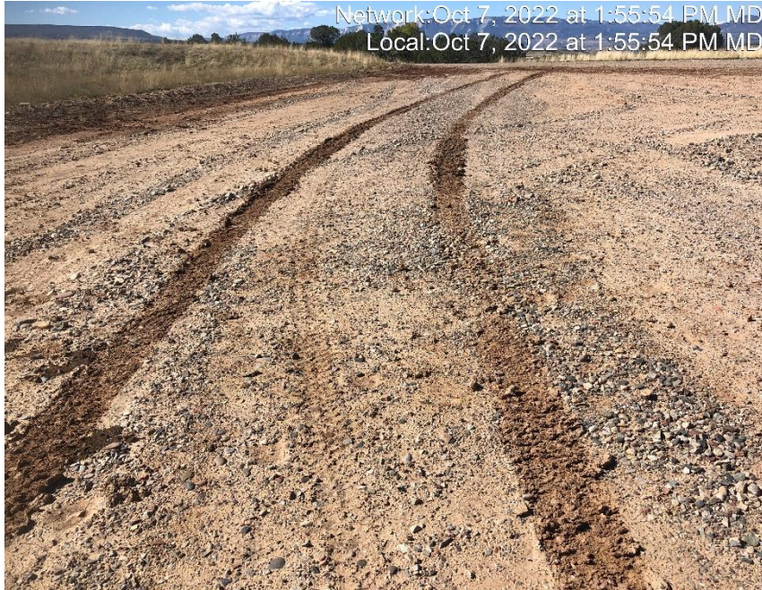
Photo #7985 Location lacks stabilization.
