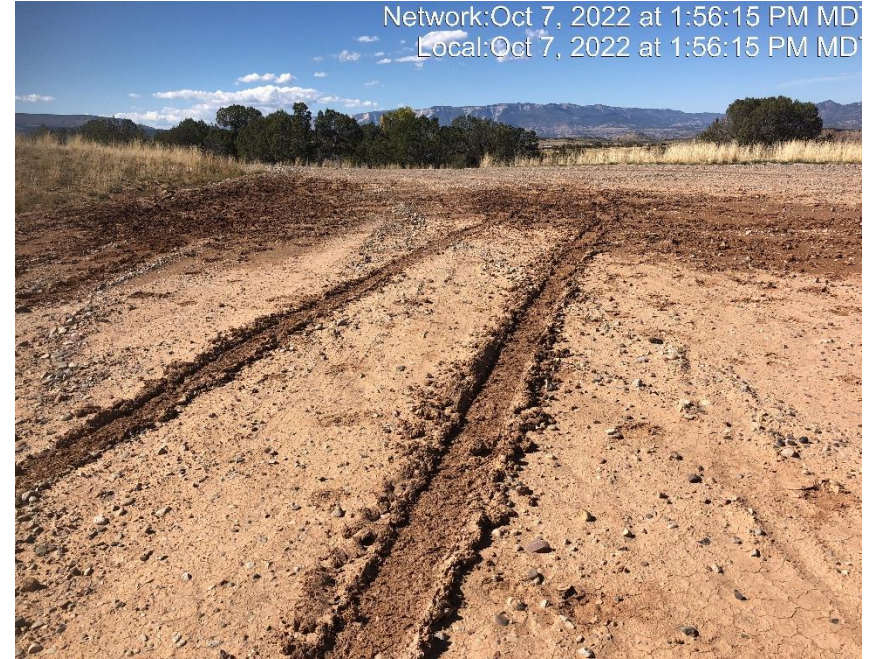
Photo #7986 Insufficient tracking BMP at entrance to location.
