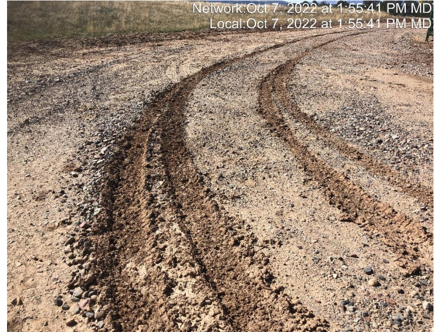
Photo #7984 Location lacks stabilization.
