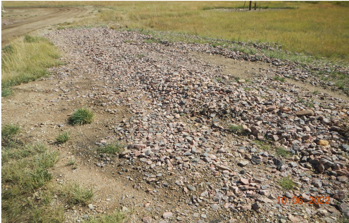
Photo 4. There is gravel debris from a pile stored on location. The leftover gravel needs to be removed. This disturbance area needs to be reclaimed.
