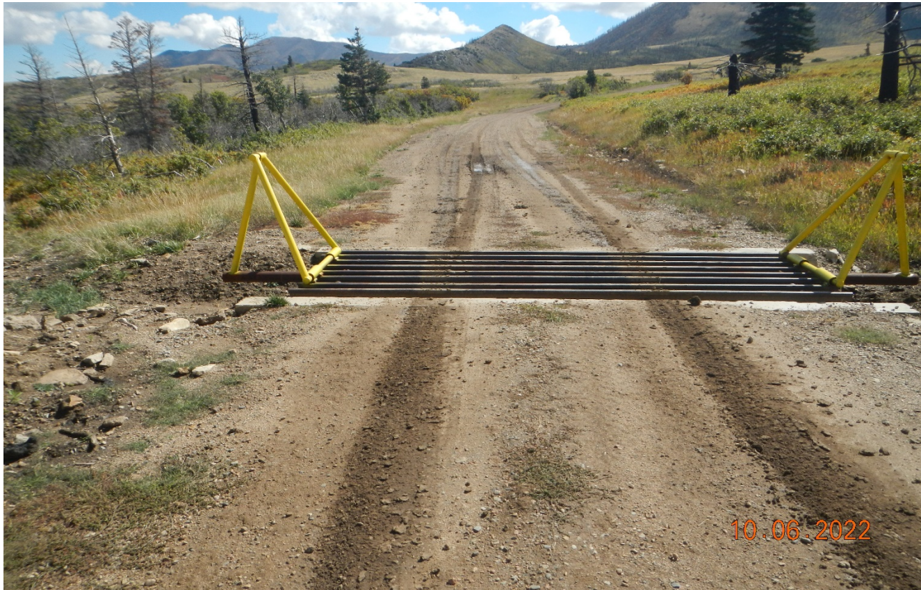
Photo 1. The cattle guard is damaged and needs to be repaired or removed.
