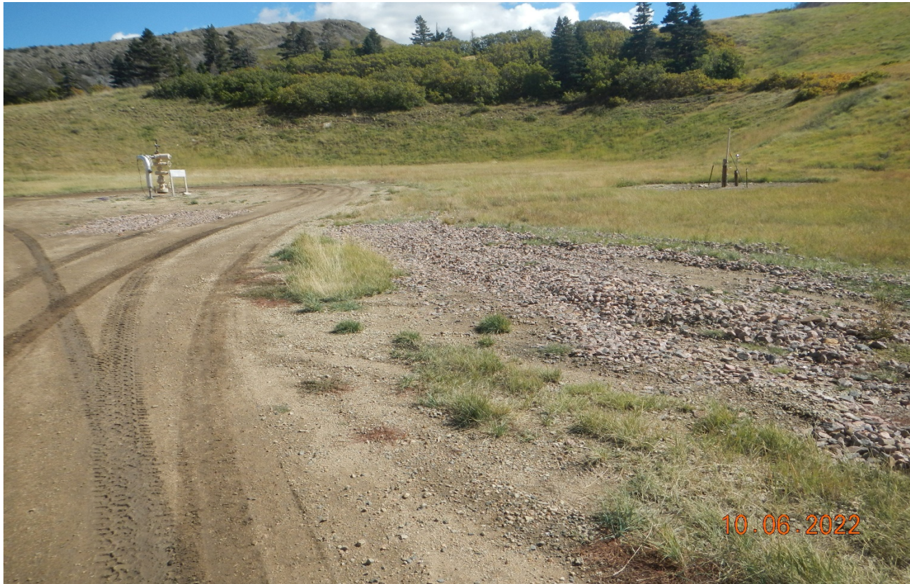
Photo 3. Facing southeast toward the well site. The gravel debris still remains and was just pushed out disturbing interim reclamation.
