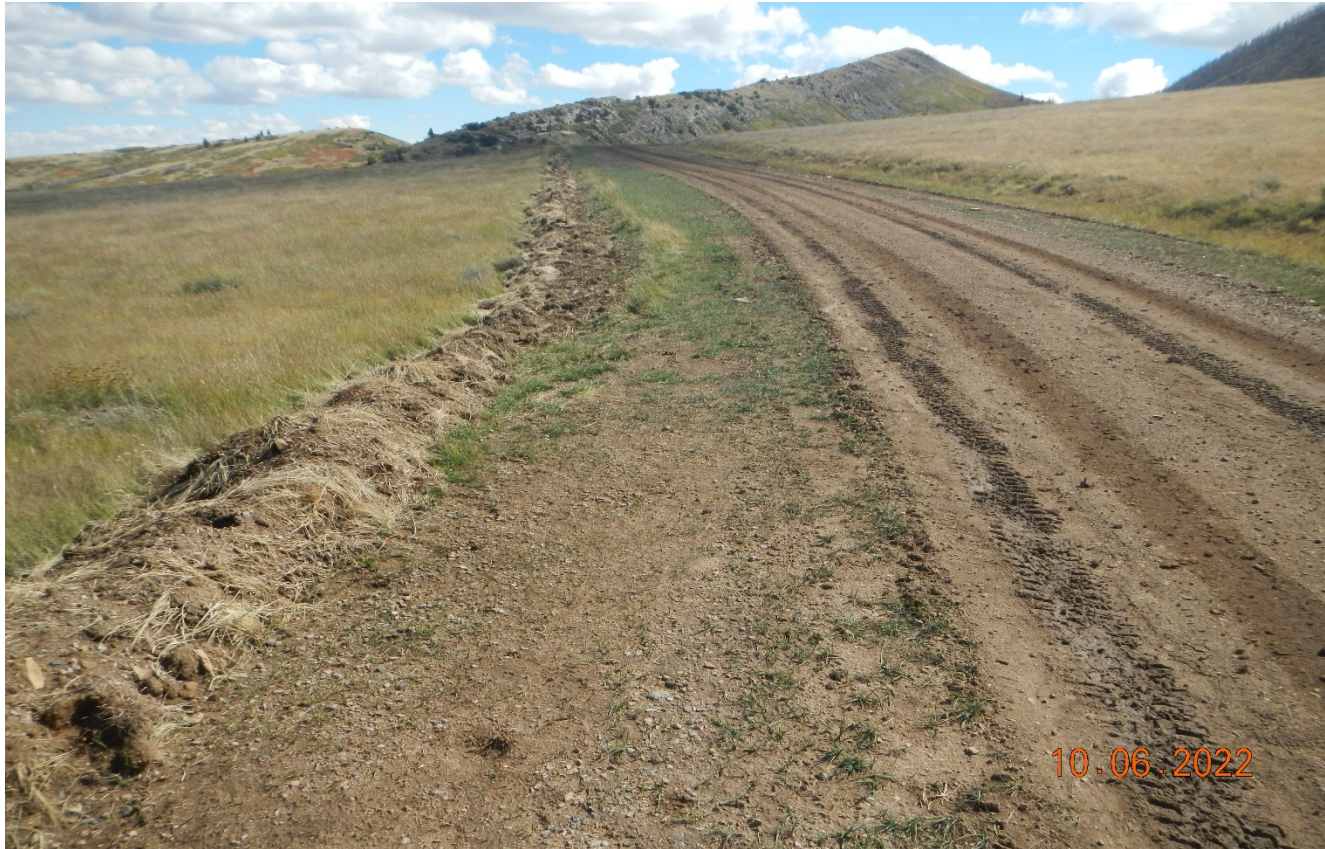
Photo 2. There has been grading performed along the road however, gravel material has been pushed off the road causing additional disturbance
