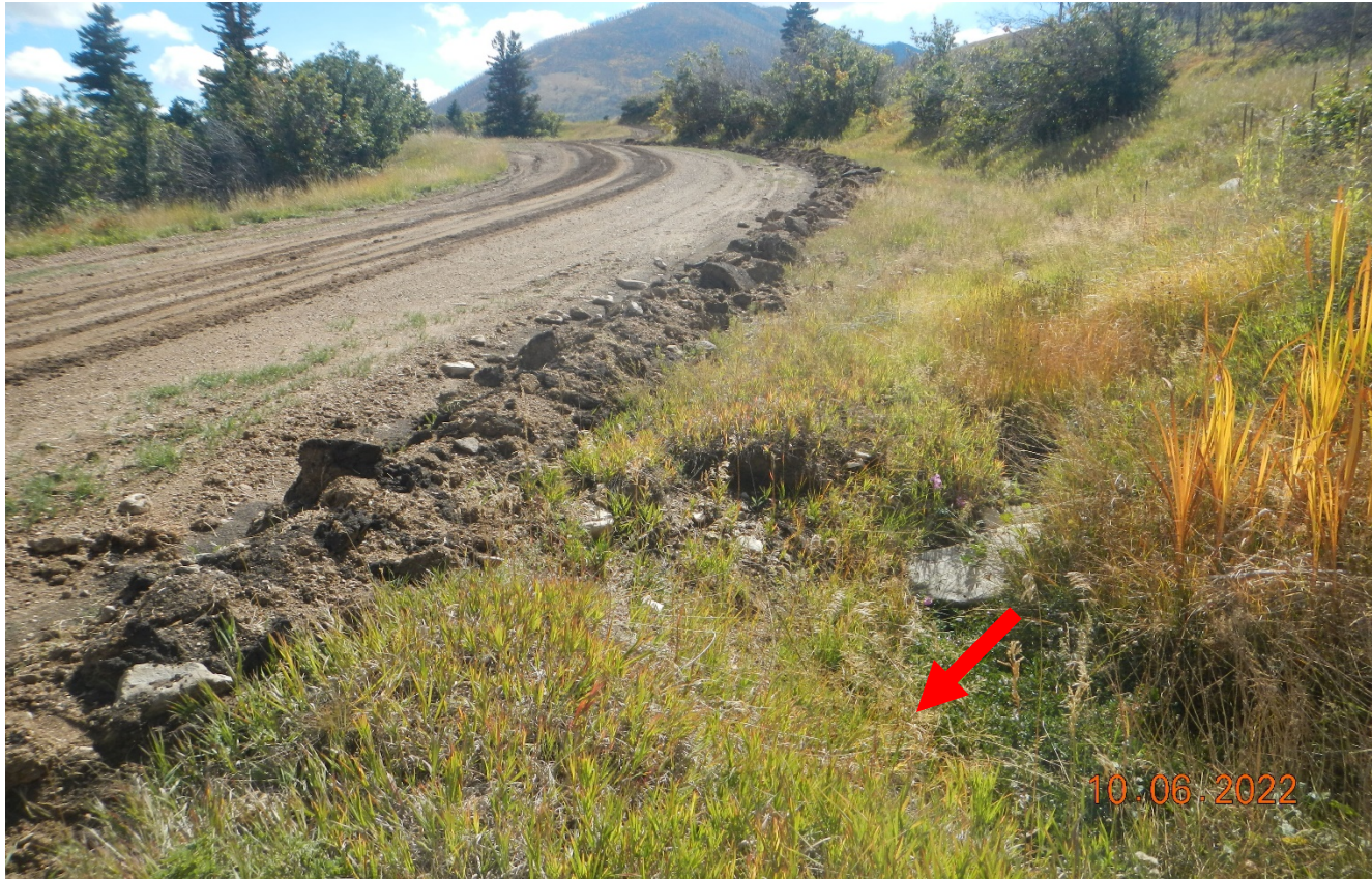
Photo 1. Facing southeast ascending the hill toward the location. There has been grading performed which has pushed gravel material to the side which is now interfering with stormwater flow to the culvert which is at the red arrow.
