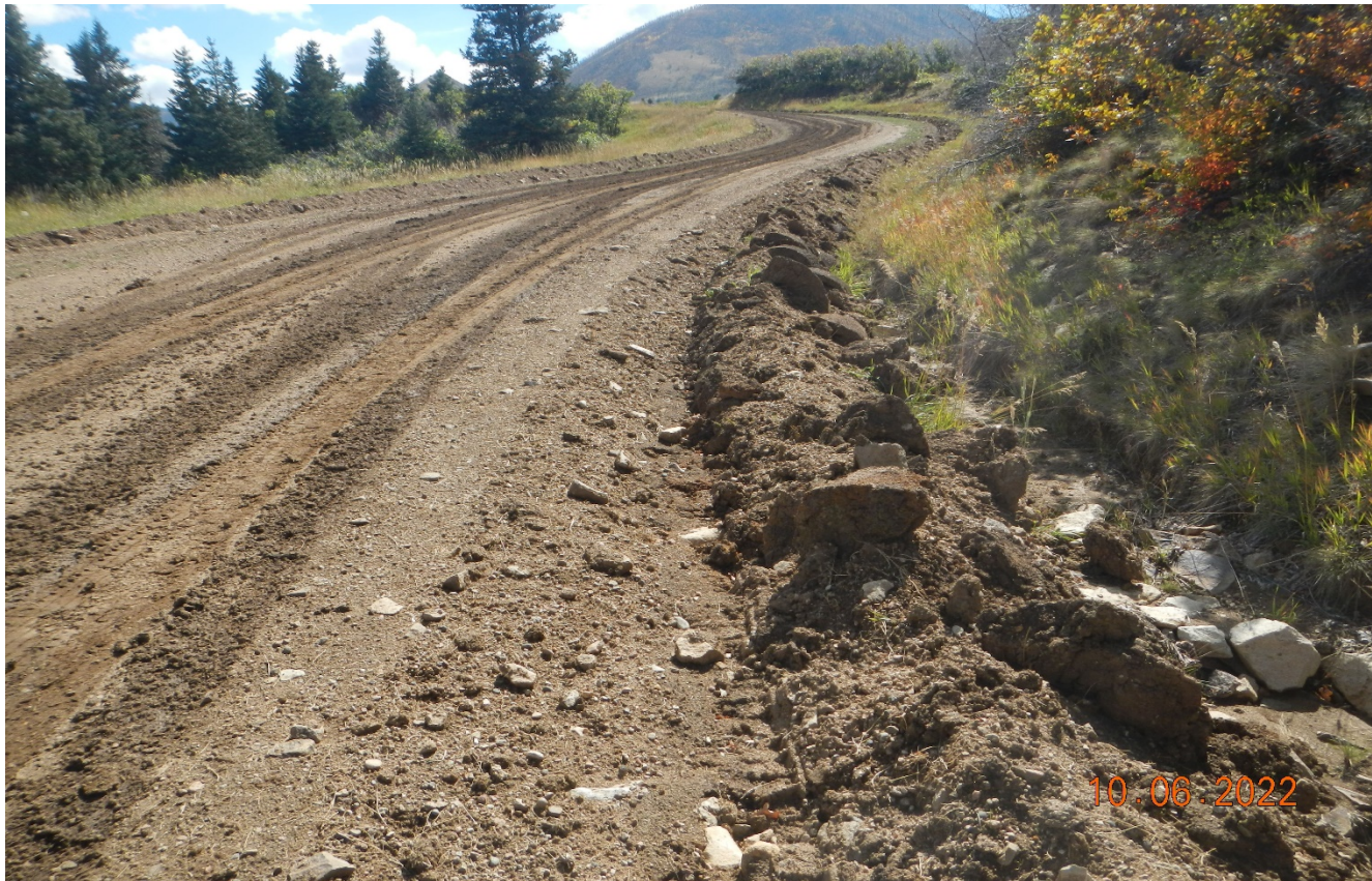
Photo 3. Facing southeast ascending the hill toward the location. There was no BMP's installed along the roadside where erosion had occurred and loose soils were pushed off the side which are susceptible to erosion.
