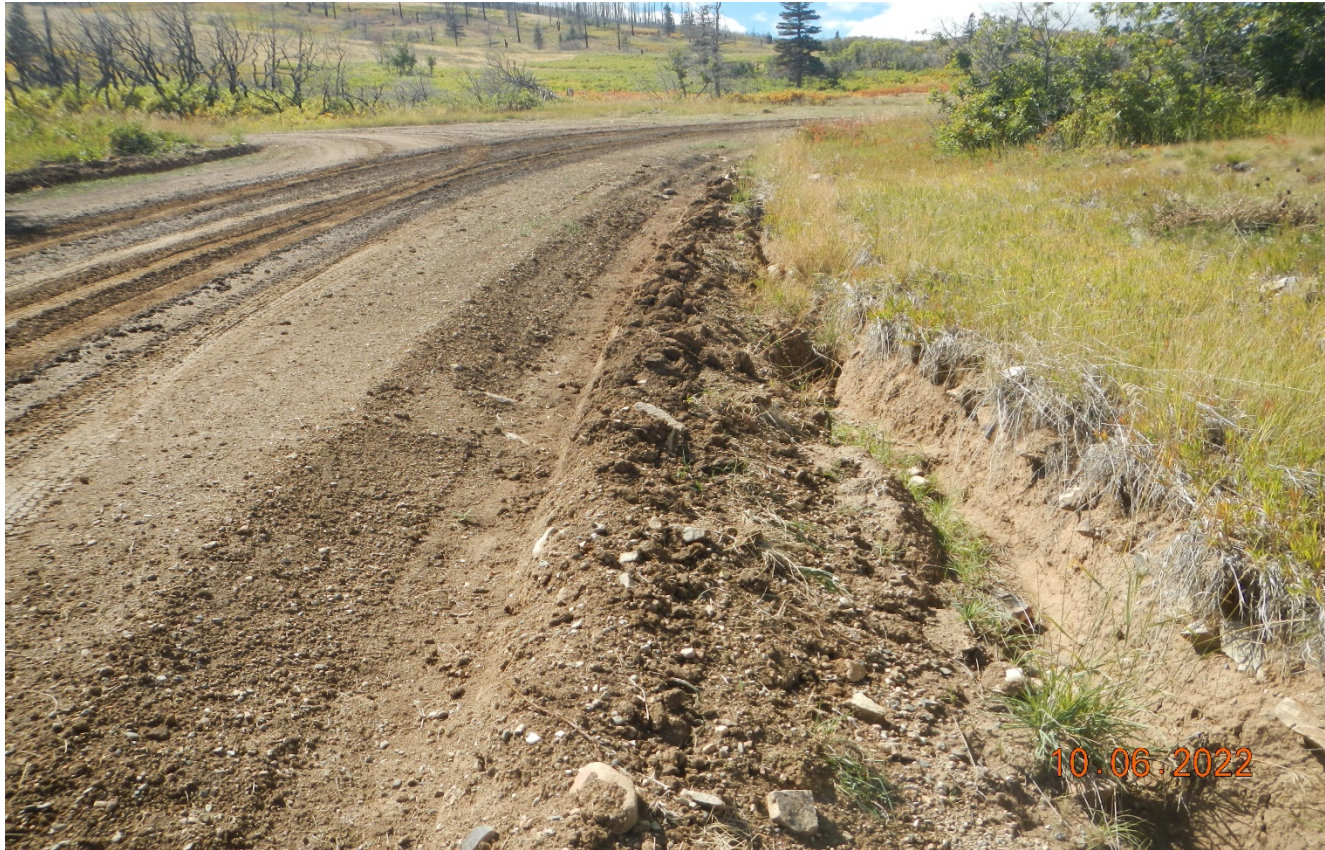
Photo 5. Further along the road is another area where erosion of the road side had occurred and loose soils have been pushed into this area. This area needs to be repaired and stabilized.
