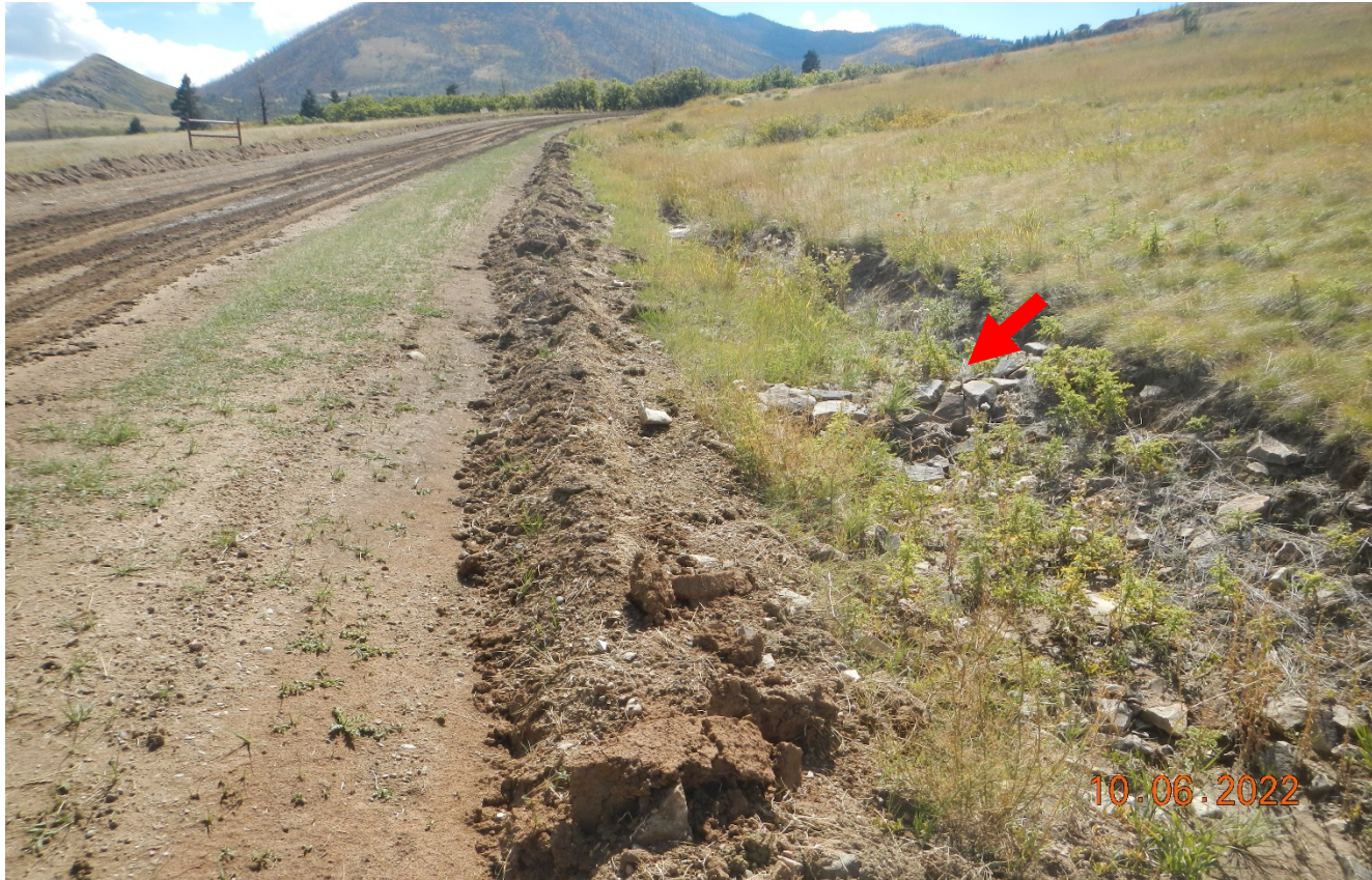
Photo 4. Facing southeast ascending the hill toward the location. There has been grading performed which has pushed gravel material to the side which is now interfering with previous BMP's. Red arrow points to rock check dam. There are also numerous noxious weeds in this area that have not been controlled.
