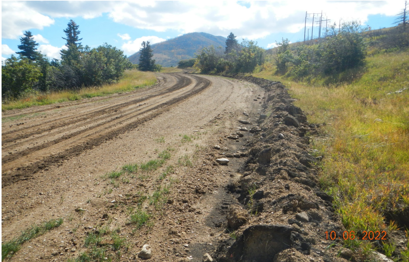
Photo 2. Facing southeast ascending the hill toward the location. The graded material is loose and susceptible to erosion. There are no BMP's to prevent erosion along this long stretch of road.
