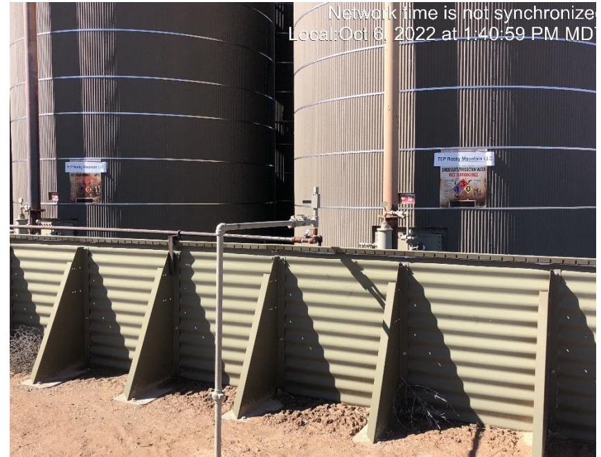
Photo #7956 Multiple tank labels weathered and not legible.
