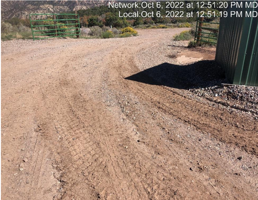
Photo #7944 Insufficient tracking BMP at entrance to location.
