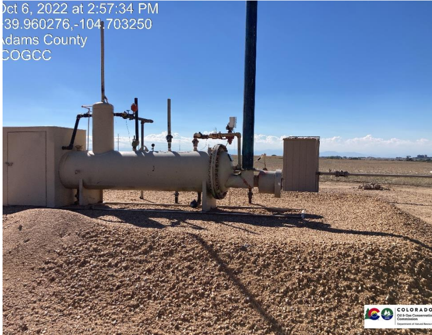
Pic 3 separator, gas meter run
