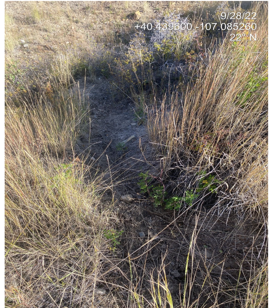
Photo 6. Photo taken from the north of the Location at the top of the fill slope shows gully erosion.
