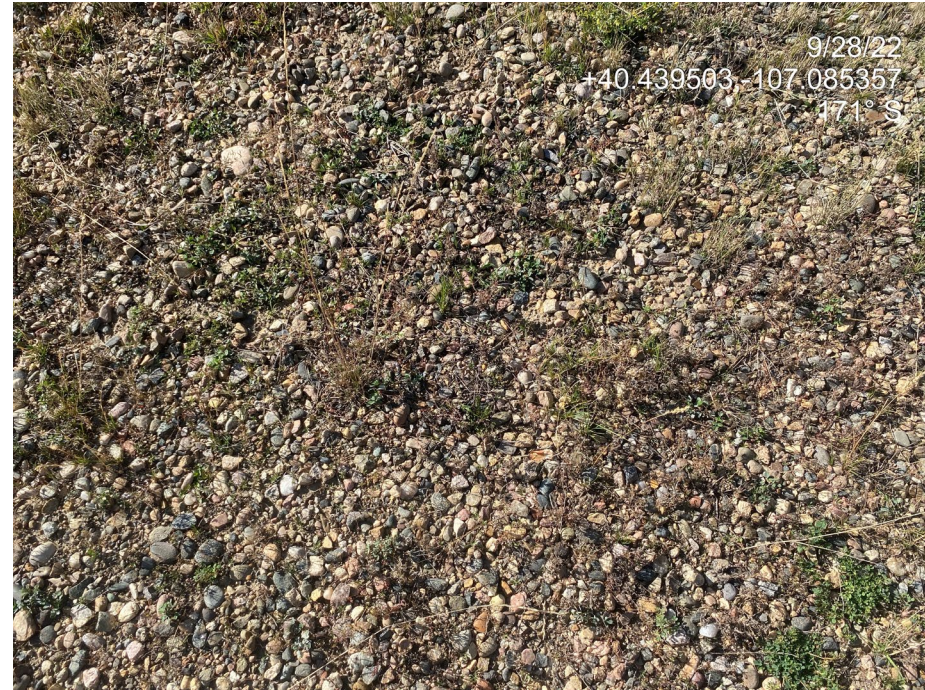
Photo 10. Photo taken from the center of the Location shows the pad surface is flat, graveled and compacted.
