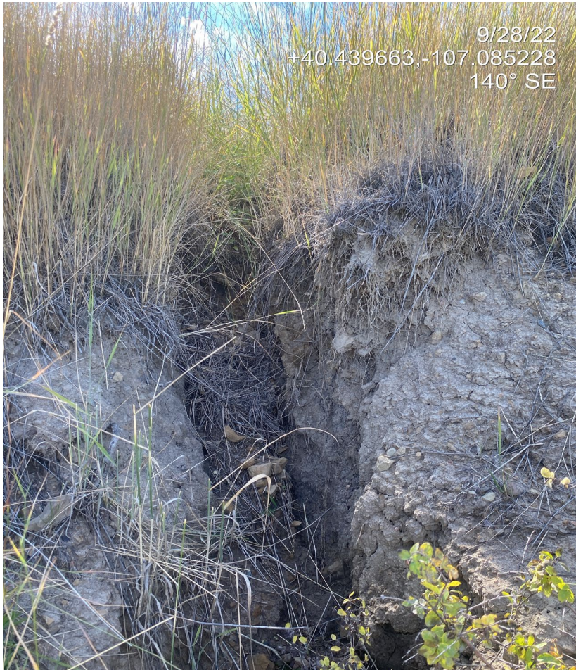
Photo 7. Photo shows gully erosion in the fill slope.
