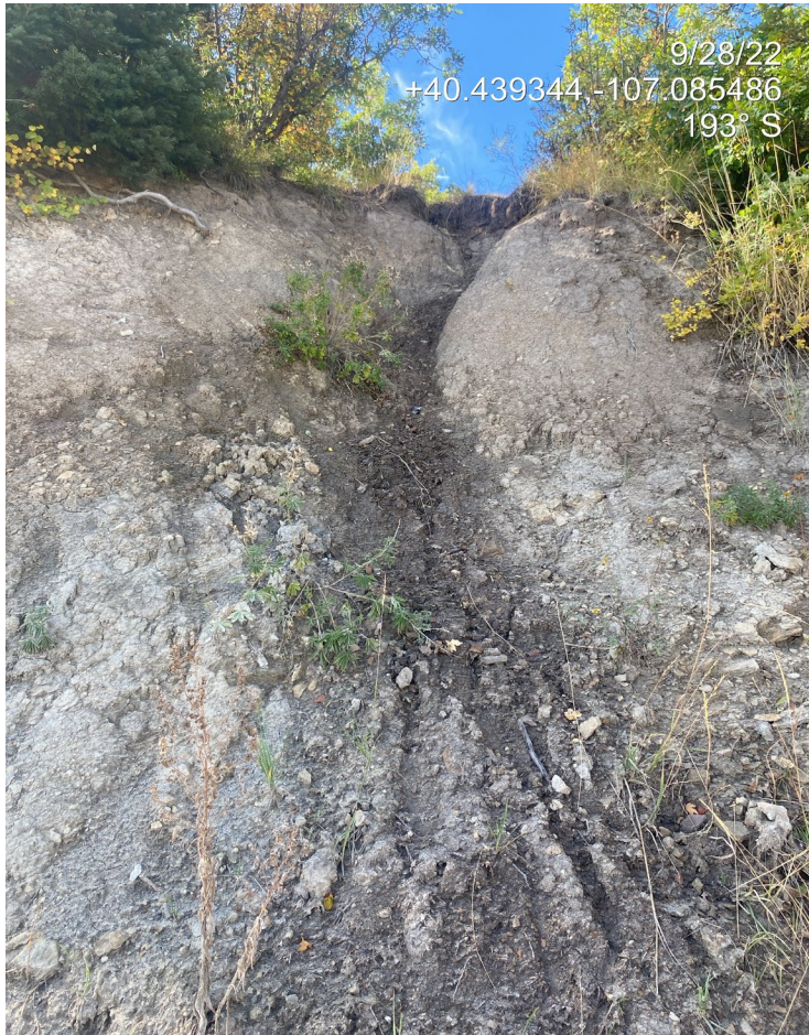
Photo 3. Photo taken from the south shows the eroding cut slope. Note undercutting and exposed roots in reference area.
