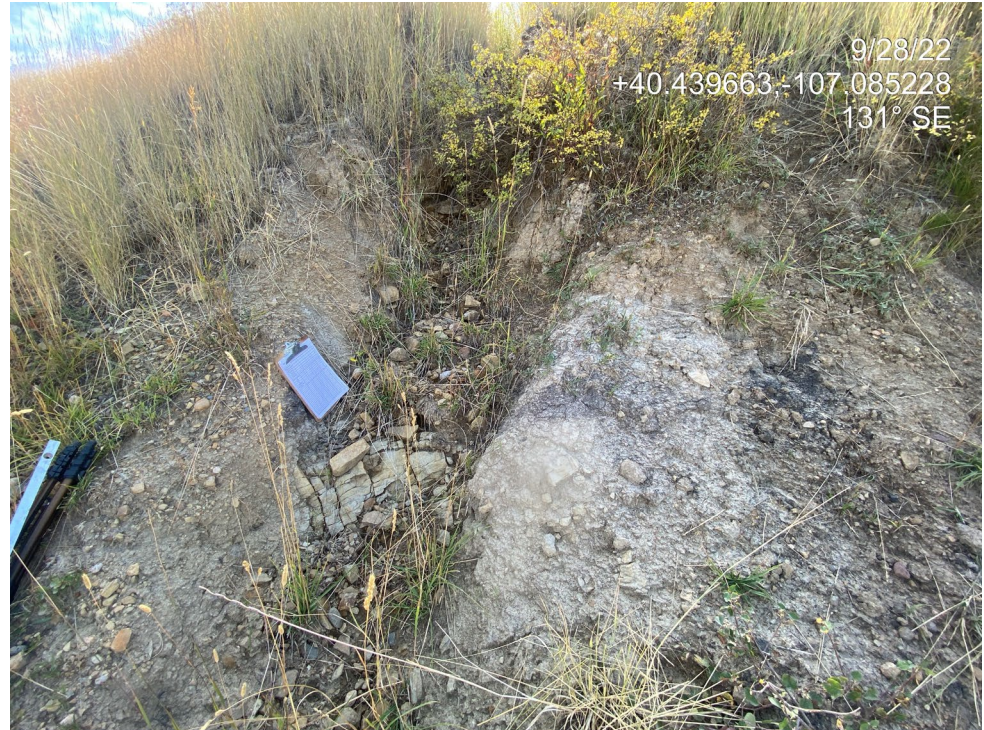
Photo 8. Photo shows gully erosion in the fill slope.
