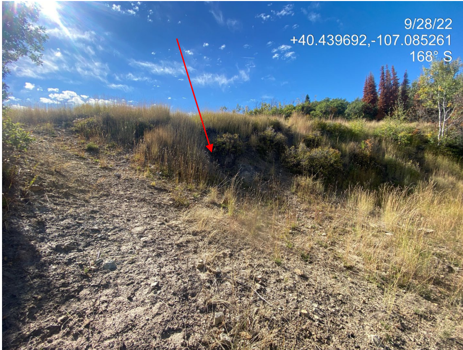
Photo 5. Photo taken from the north of the Location at the base of the fill slope. The red arrow indicates where gully erosion is occurring.
