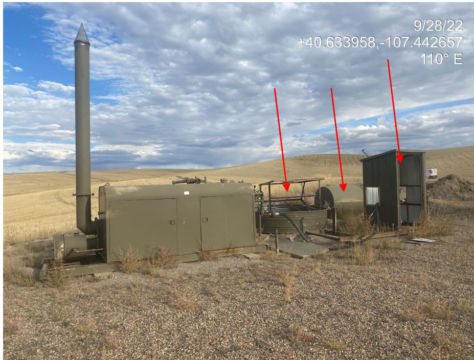
Photo 2. Photo shows a meter run with no equipment and a knocked over tank. Equipment is now debris.
