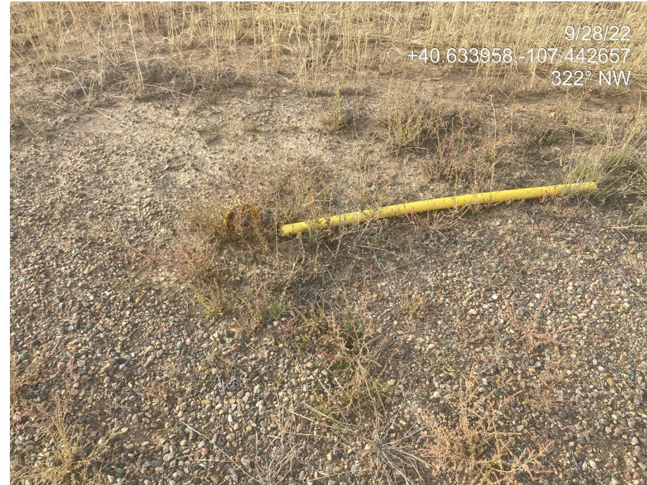
Photo 7. Photo shows an anchor marker in disrepair.
