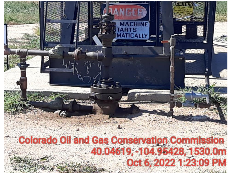
Photo 2 Stained soil around well head.
