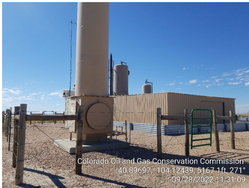
Photo 1 – ECD and Heater Treater
