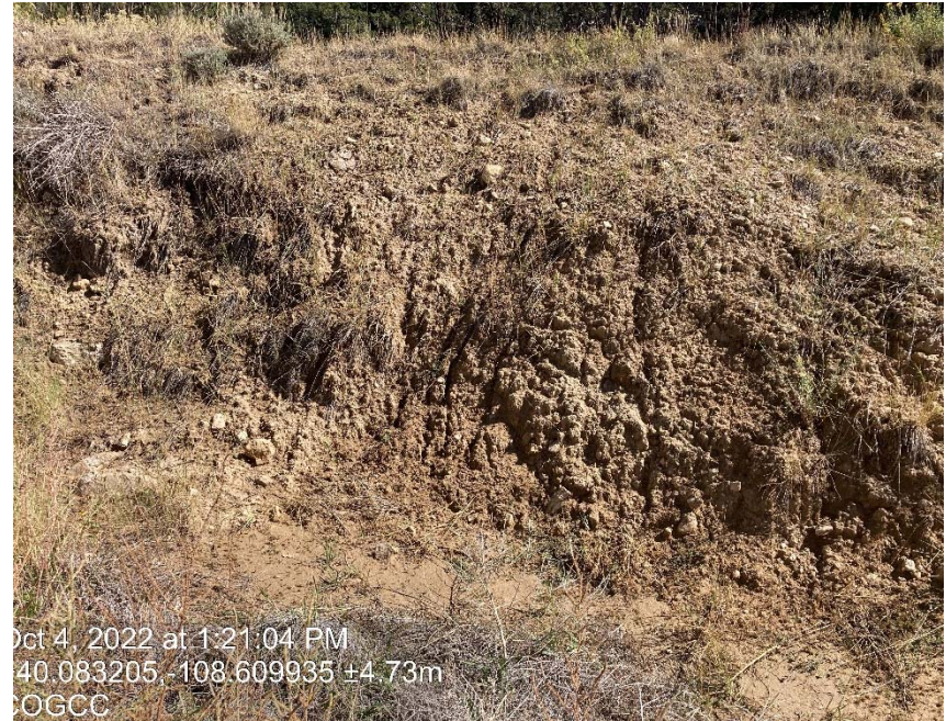
Cut slope shows signs of erosion and lack of stabilization
