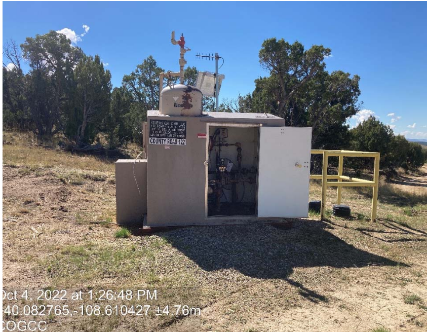
Location and lacking operator emergency number
