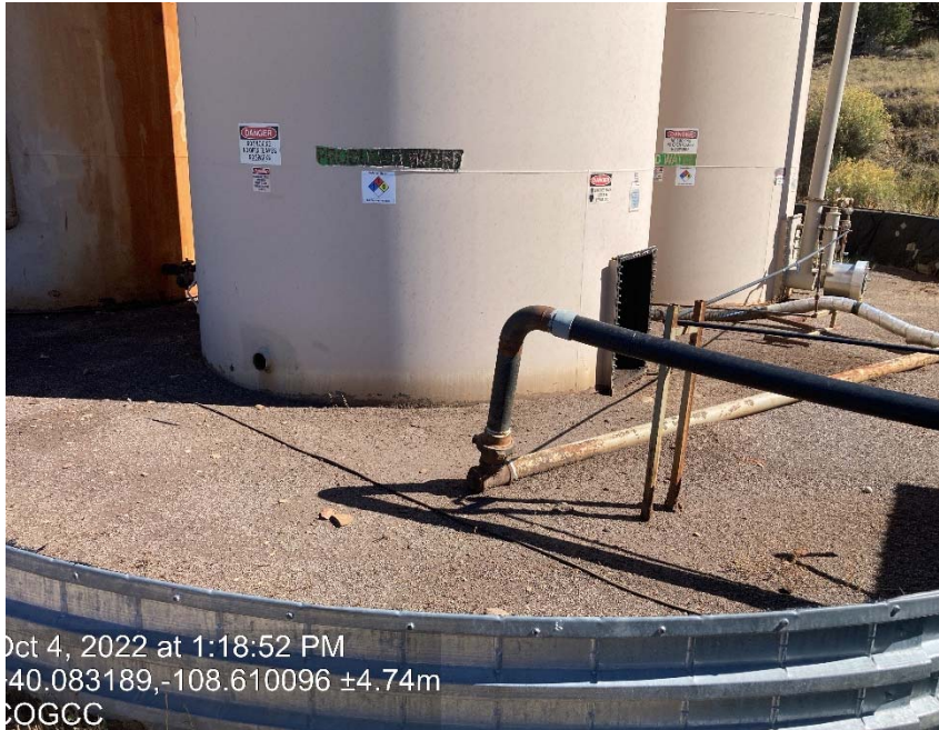
Tanks lacking proper labeling and open man way
