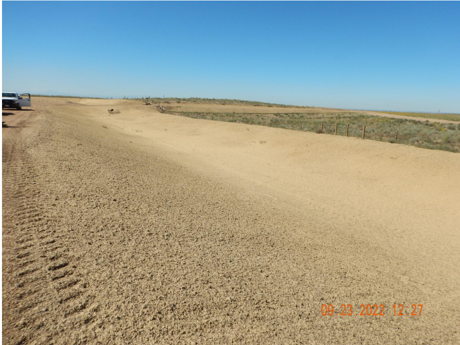
Photo 1. Photo taken from the northern location, facing West. Photo illustrates stormwater erosion repairs have been completed.
