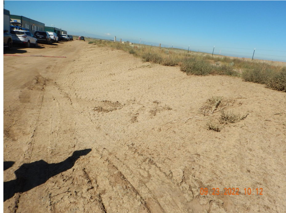
Photo 2. Photo taken from the northeastern location, facing West. Photo illustrates stormwater erosion repairs have been completed.
