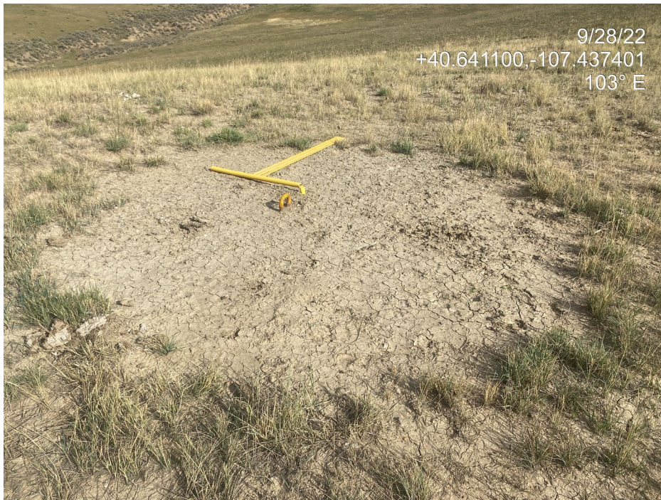
Photo 5. Photo shows an anchor marker in disrepair.
