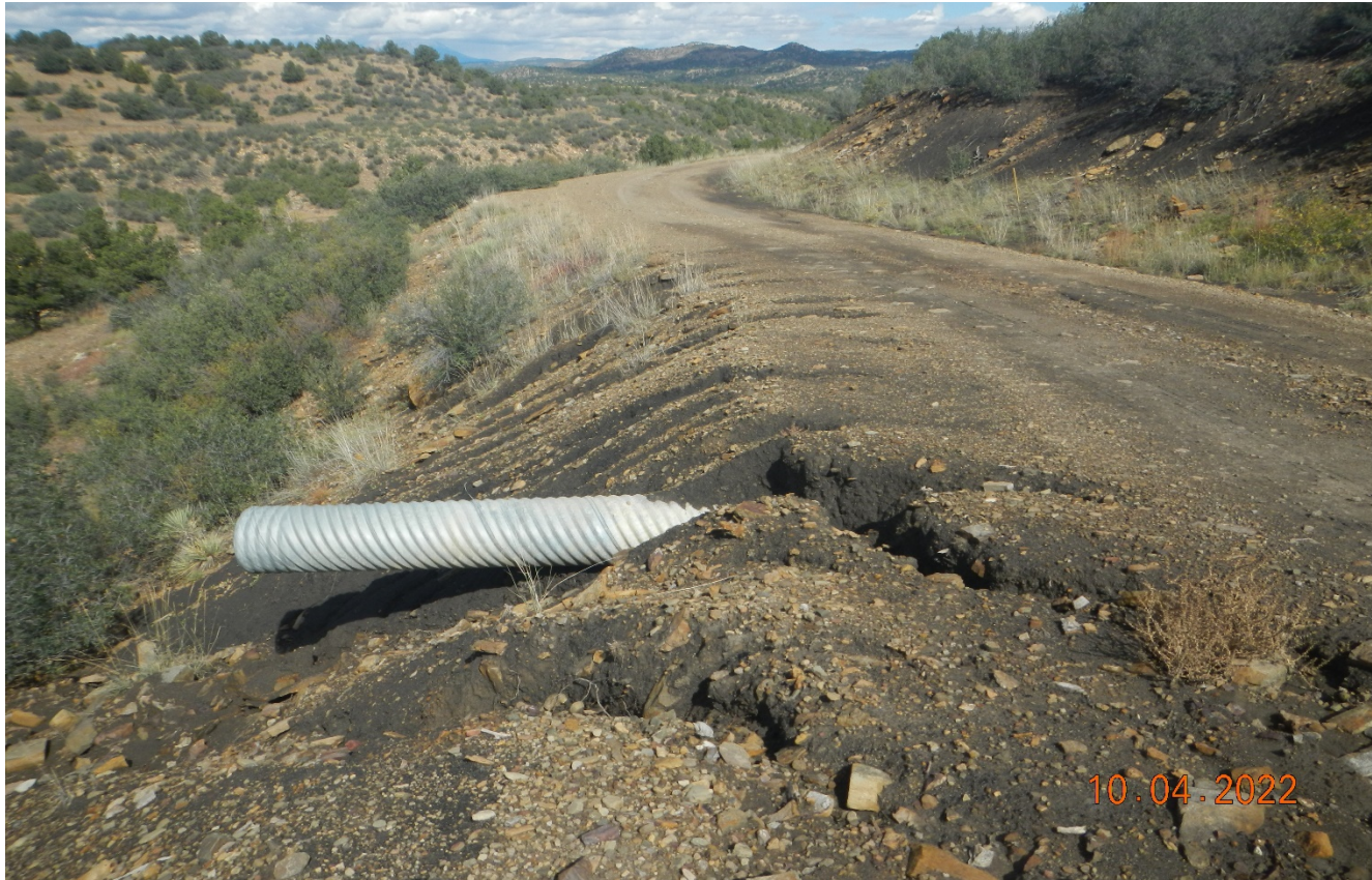
Photo 2. There is erosion occurring across the road and at the culvert outlet.
