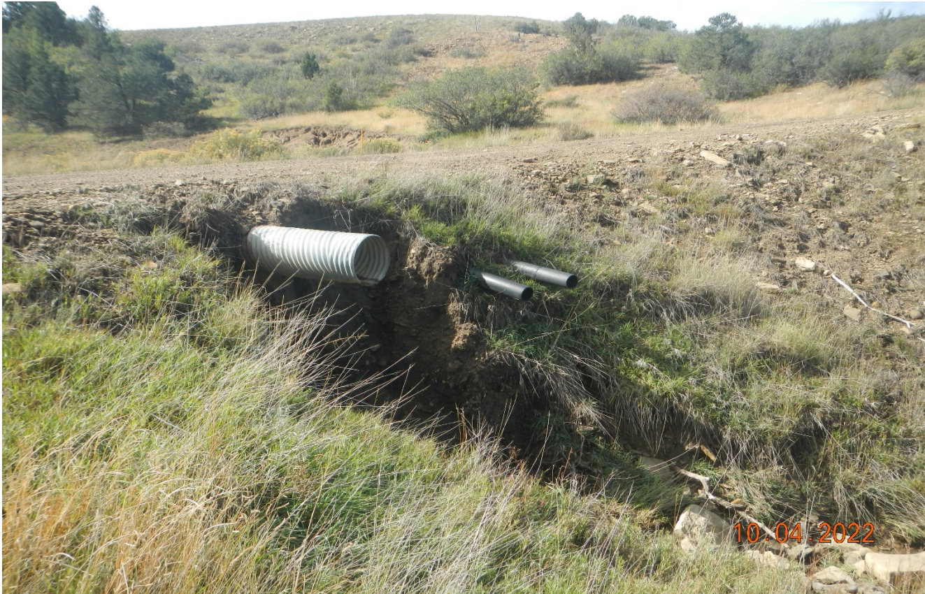
Photo 1. The culvert outlet at the drainage crossing has eroded and has no outlet protection.
