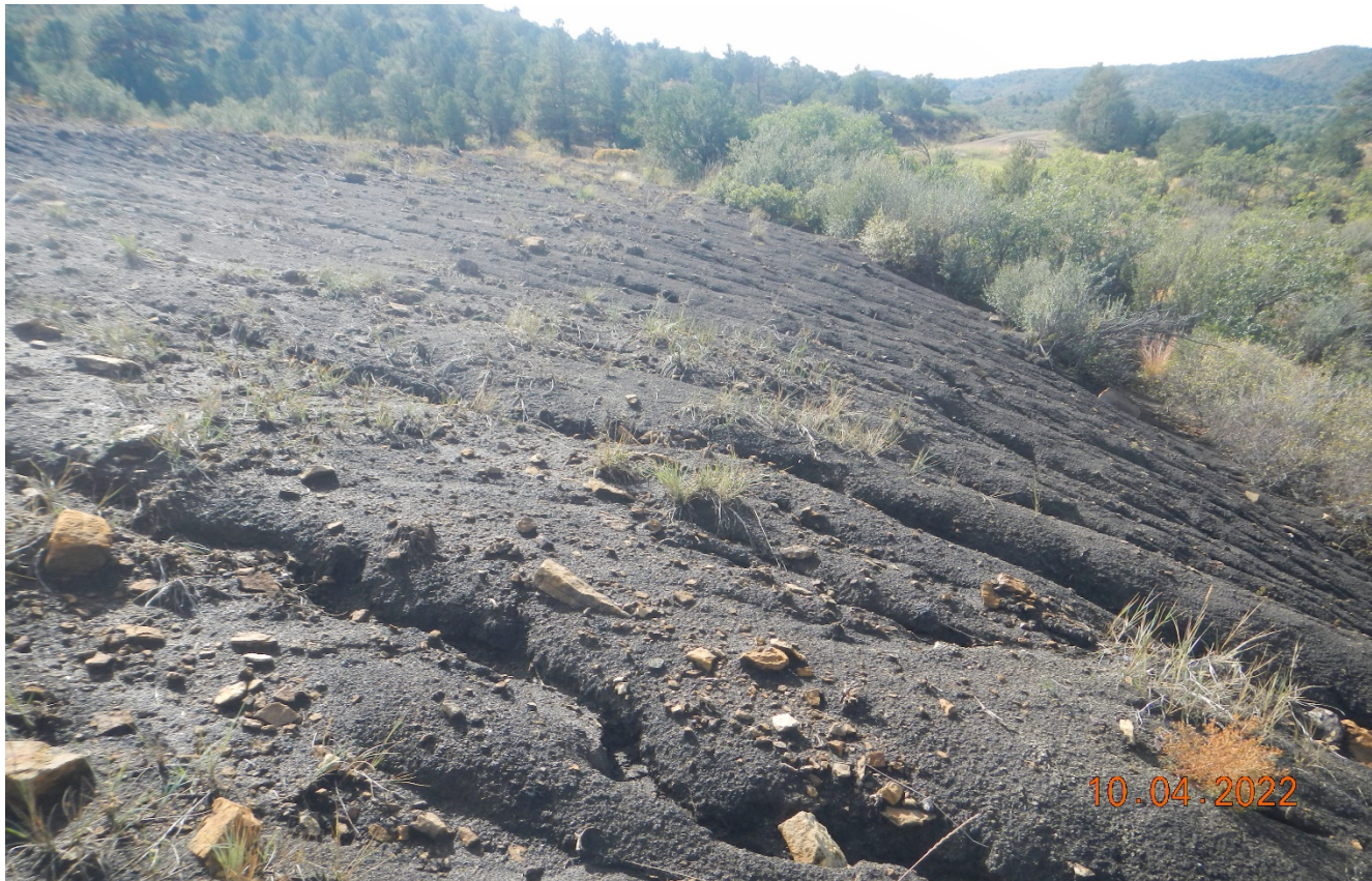
Photo 4. There is erosion along the fill slope which needs additional BMP's
