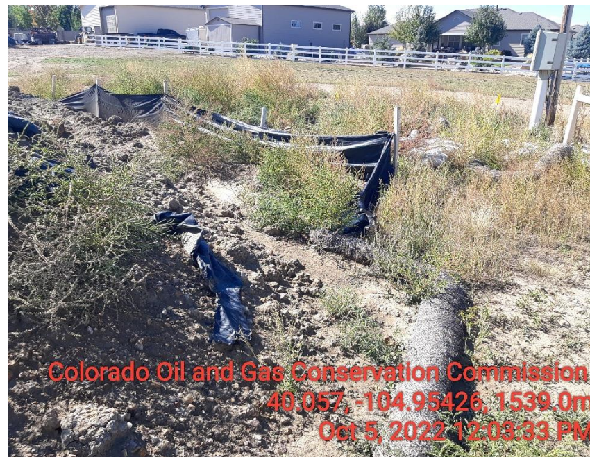
Photo 8 Inadequate stockpile BMP. BMP sediment loaded.
