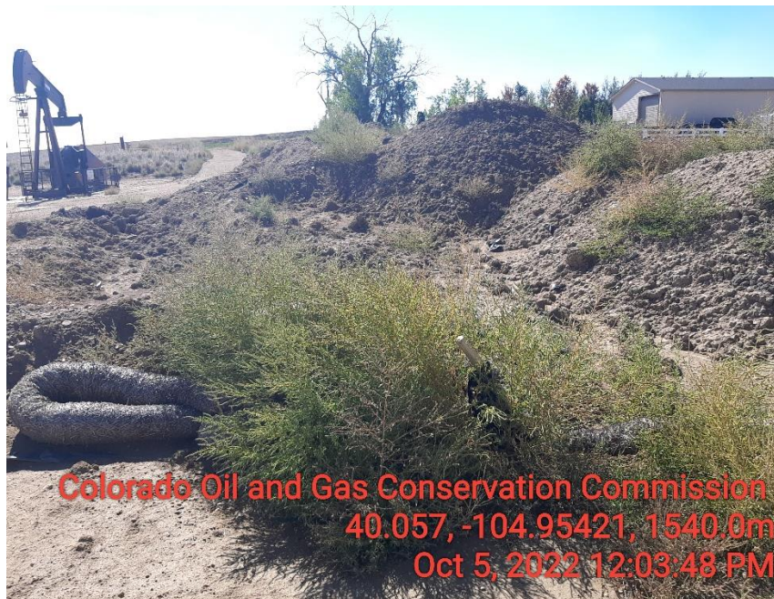
Photo 9 Inadequate stockpile BMP No liner underneath contaminated soil stock pile
