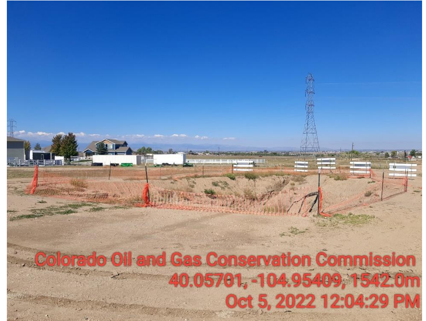
Photo 12 inadequate fencing around open excavation. Homes are approx..150 feet to the west. No BMP in place to control run on of water into excavation.
