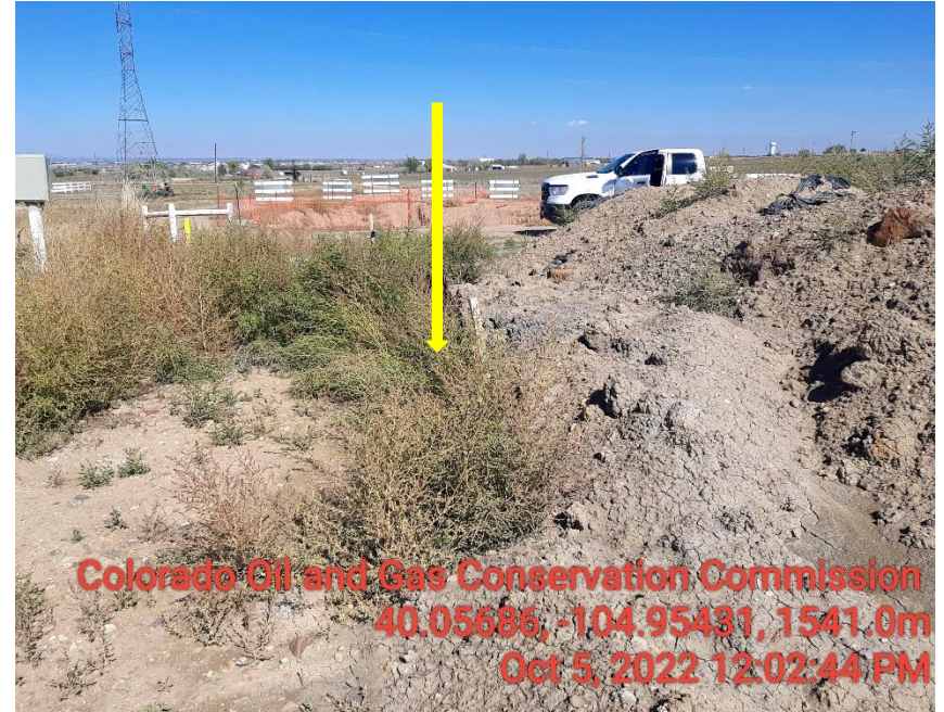
Photo 6 contaminated stock pile BMP overloaded and sediment leaving BMP
