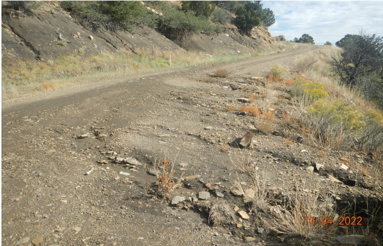
Photo 1. Facing northeast along the access road. There is erosion occurring across the road in this area.
