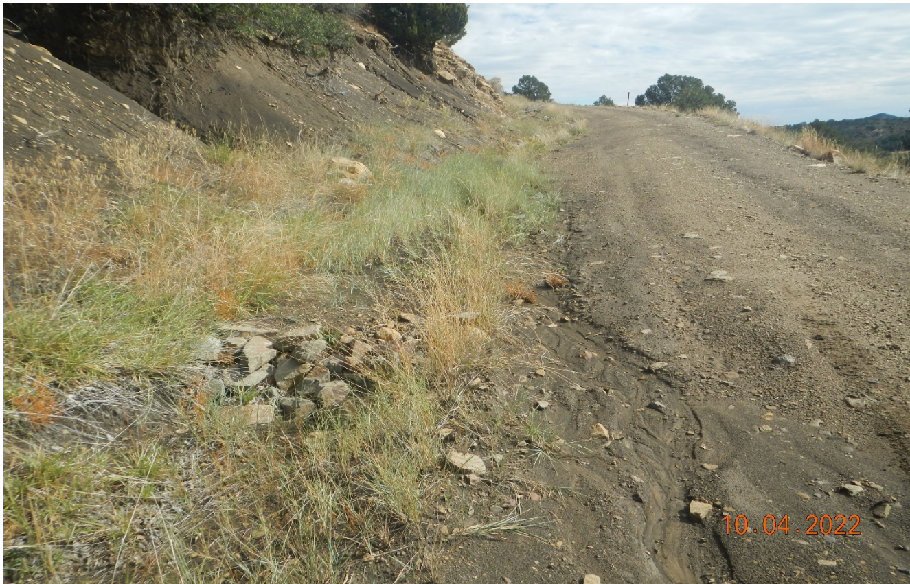
Photo 2. Facing northeast along the access road to the well site. The check dams have filled in with sediment causing stormwater to flow around onto the road.
