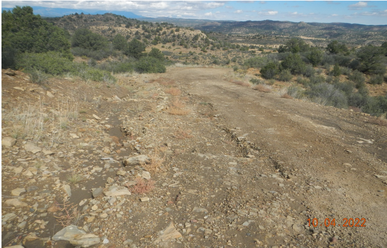
Photo 2. Facing northwest along the access road to the well site. There is erosion occurring down the road and rock check dams have filled in with sediment
