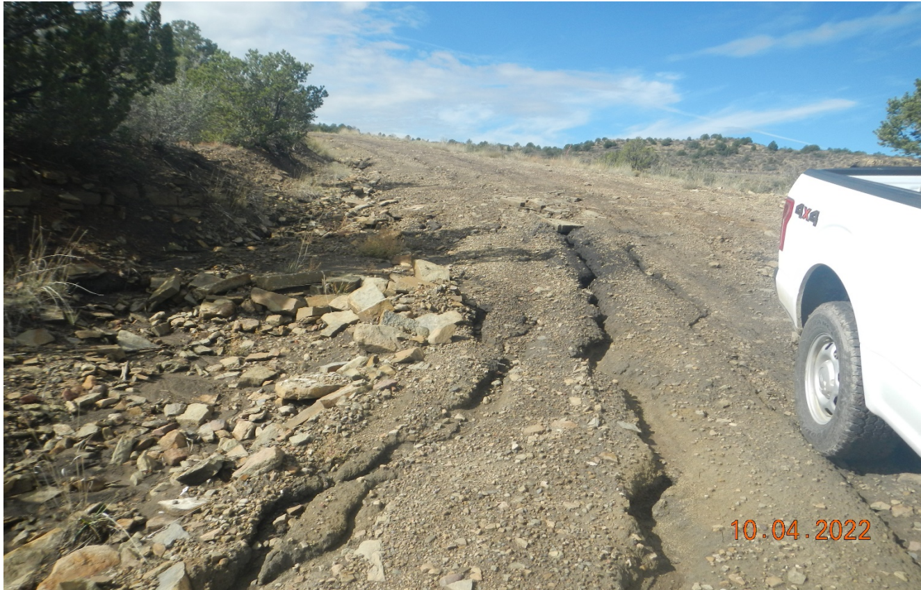
Photo 3. Facing back southwest along the access road to the well site. There is erosion occurring down the road and rock check dams have filled in with sediment.
