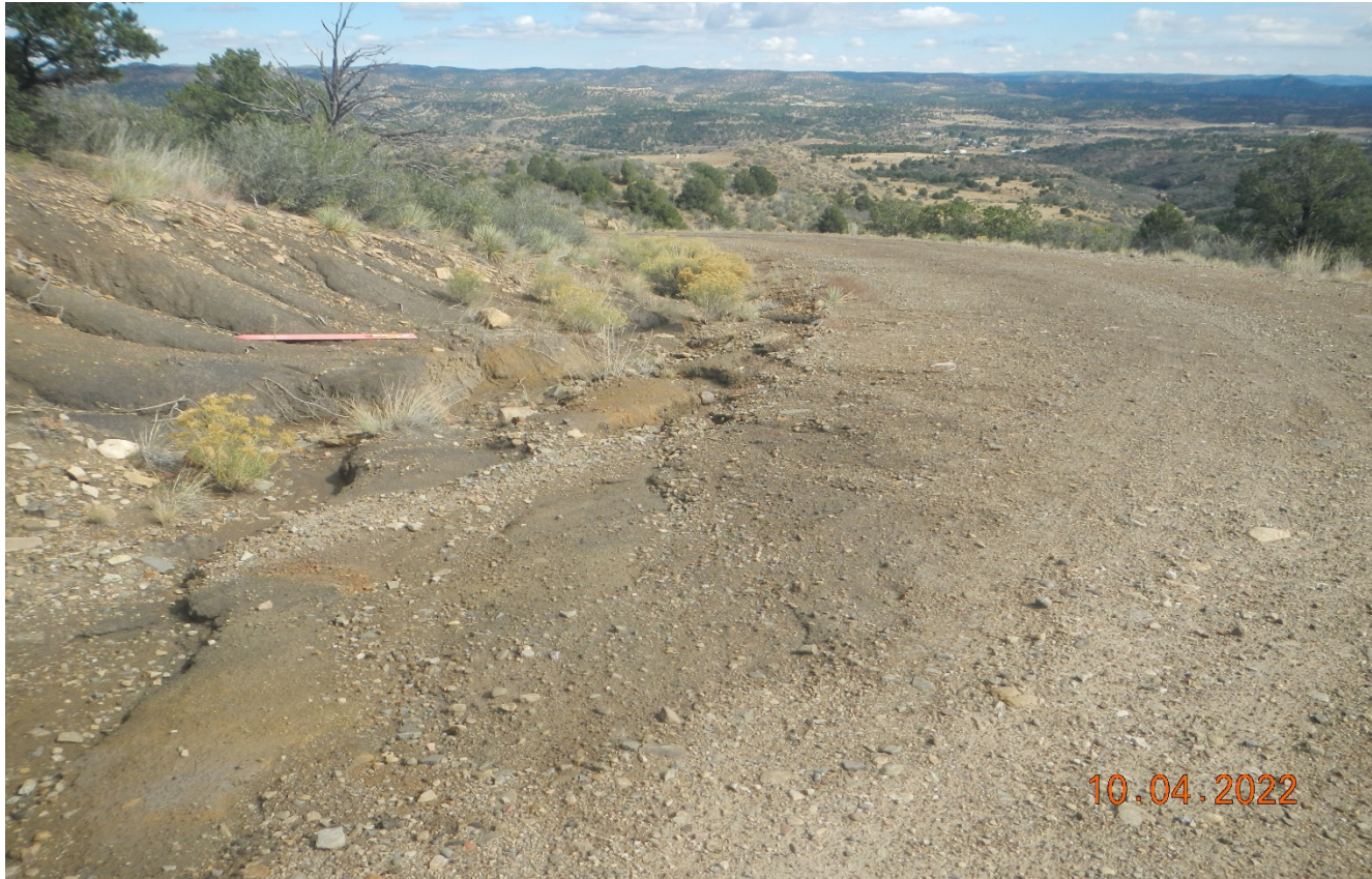
Photo 1. Facing north toward the beginning of the access road. There is erosion along the road side that needs to be repaired.
