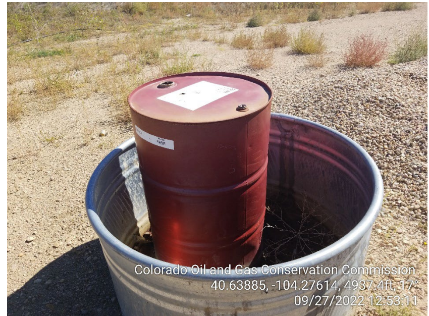
Photo 6 – Secondary Containment – Weildlife Netting is missing
