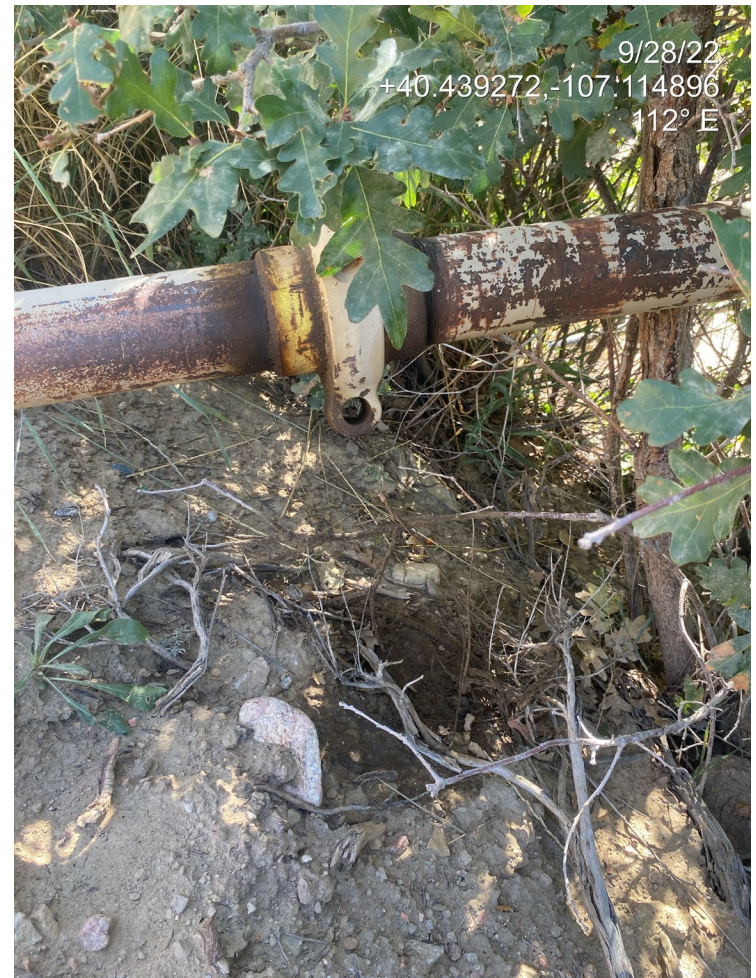
Photo 7. Photo shows stained soil beneath a load line pipe.
