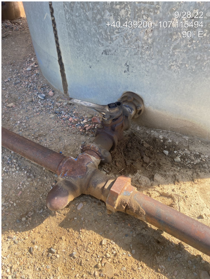
Photo 6. Photo shows stained soil beneath a tank valve
