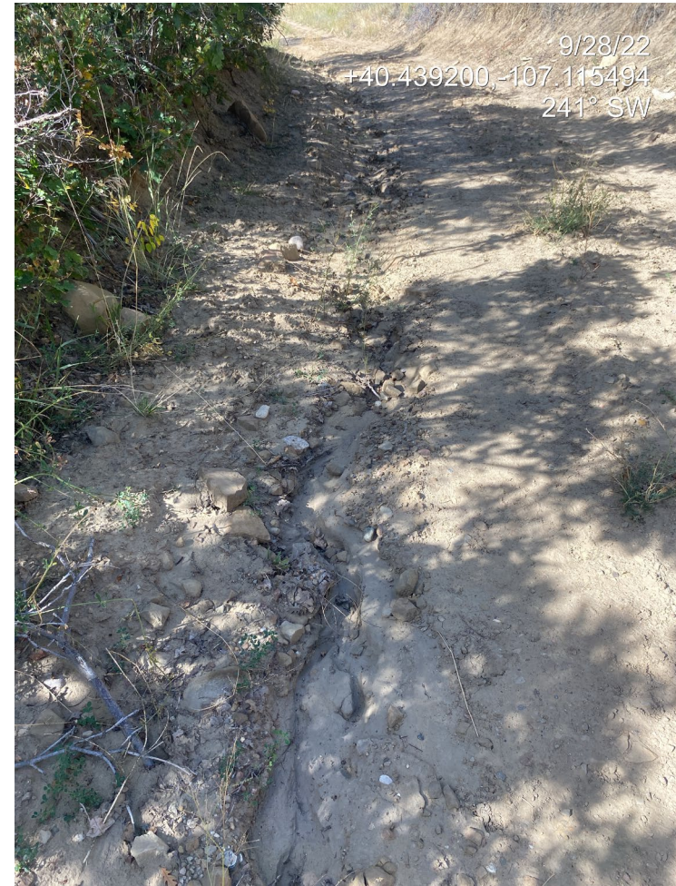
Photo 8. Photos show erosion occurring on the access road at the west of the Location.
