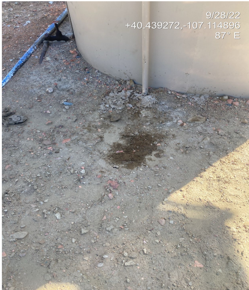
Photo 4. Photo shows stained soil within the tank secondary containment.
