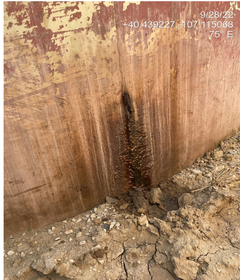
Photo 5. Photo shows where the contents of a tank appears to be weeping from the side of the tank.
