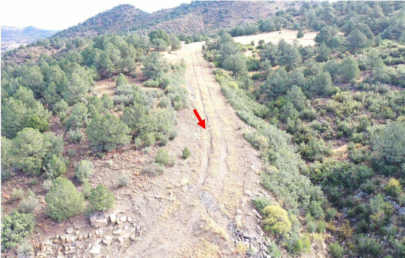
Photo 10. Facing northeast toward the access road which was not recontoured and reclaimed. The access road switches back and dead ends at the location. There is erosion occurring down the road shown at red arrow.
