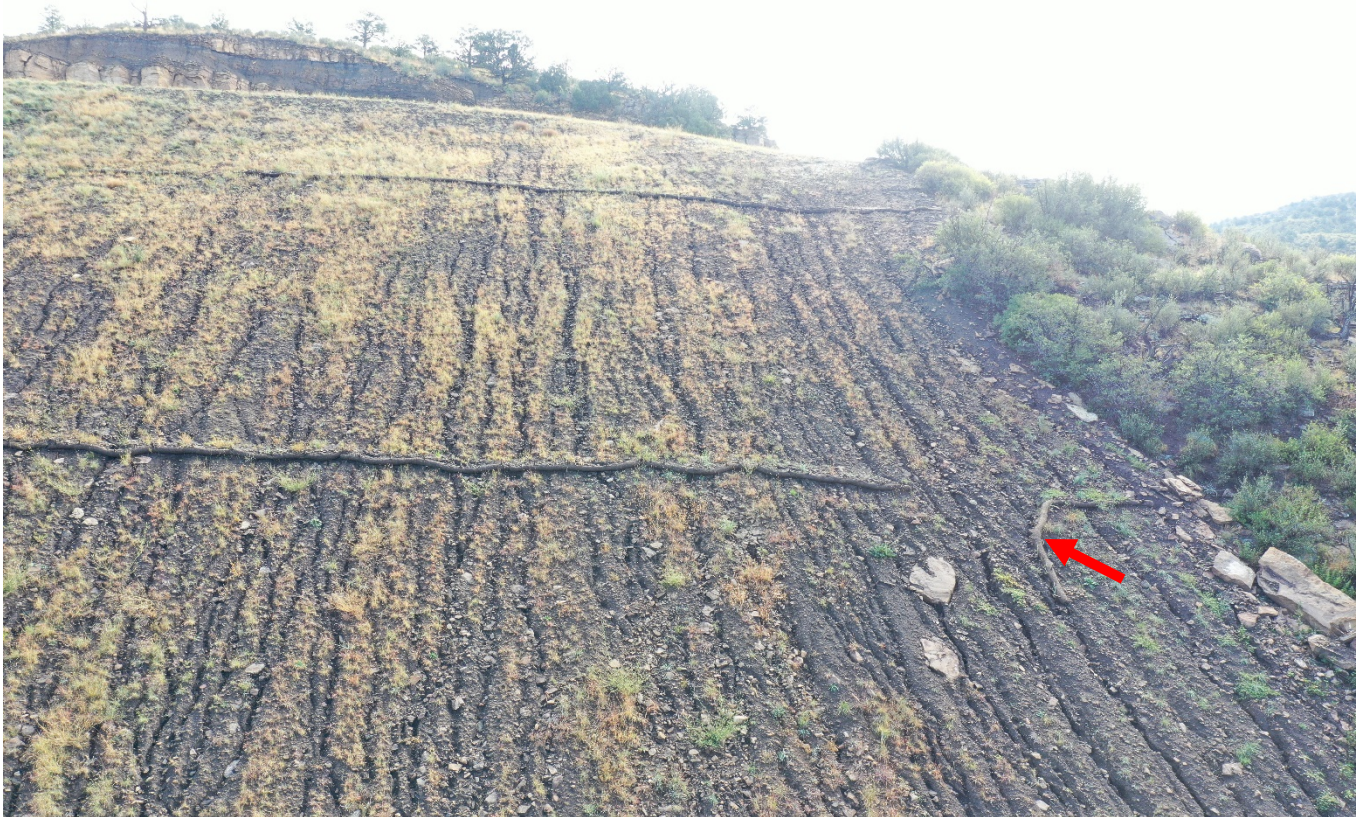
Photo 4. The straw wattles along the cut slope are displaced and not maintained. Red arrow points to the same displaced wattle observed during the previous inspection last year. Previous corrective action was not performed.
