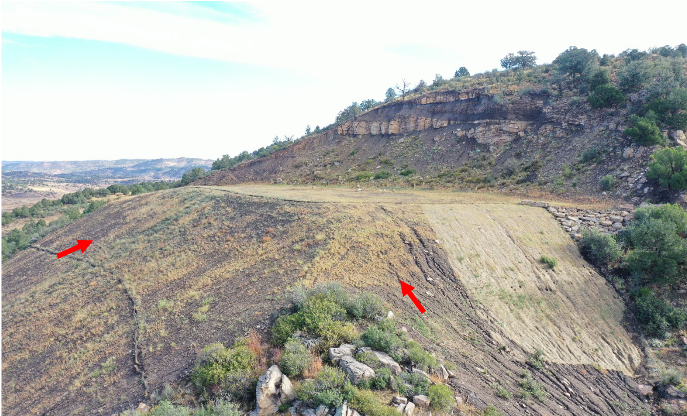
Photo 6. Facing north toward the location which was not recontoured per the rules. The red arrows point to fill material which could have been safely placed back to original contour which would have reduced the grade of the slope. Typically excavators are used to pull material back into the cut slope.
