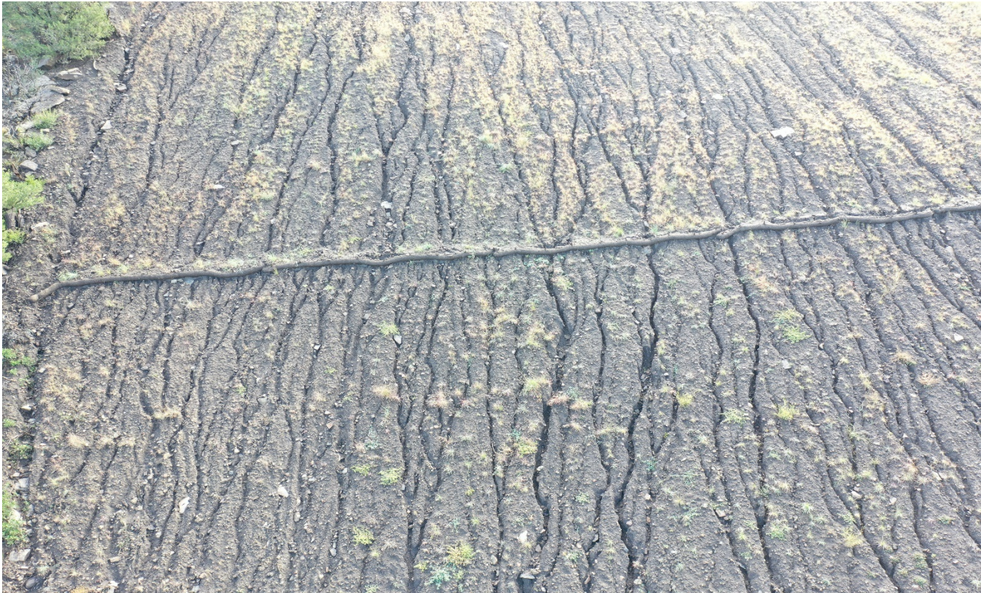
Photo 3. Facing closer to the fill slope shows the rilling erosion that has occurred. The wattles are not maintained and have filled in with sediment. Rilling erosion continues to occur underneath the wattles and down the slope.
