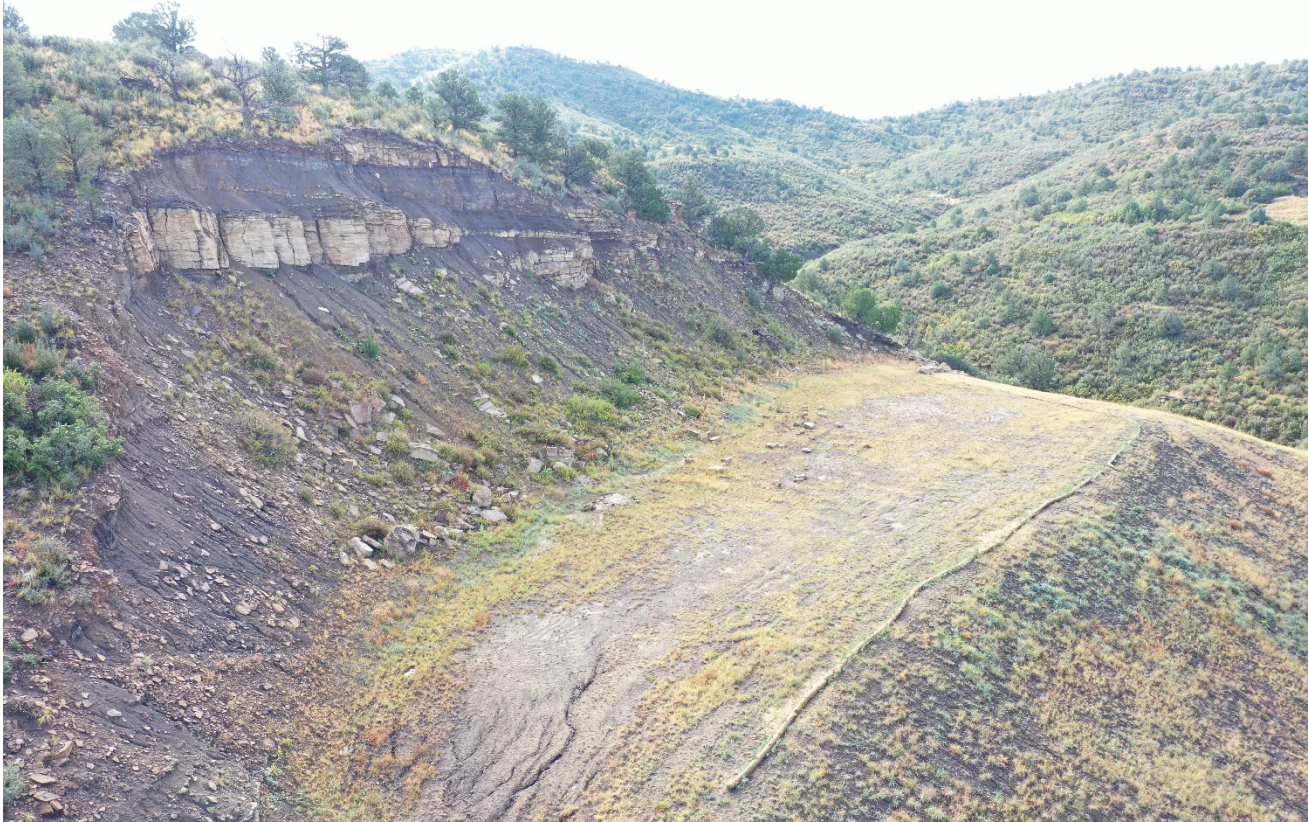
Photo 8. Facing southeast toward the location. A vertical unstable cut slope still remains and is not stabilized. The fill slope material was not resloped back to the original contour.
