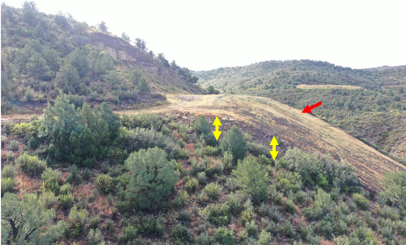
Photo 7. Facing southeast toward the location which was not recontoured per the rules. The red arrow point to fill material which could have been pushed back to original contour. The yellow arrows show fill material which is about 20ft. from the original grade.
