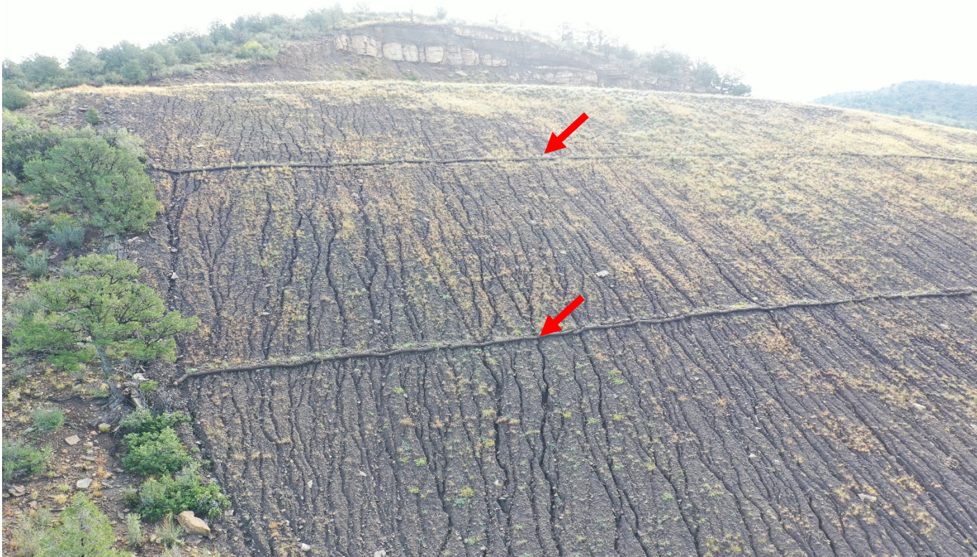
Photo 2. Facing east toward the fill slope. Stormwater controls were not sufficient and there is significant erosion along fill slope. The red arrows point to the two rows of wattles that are filled in with sediment and have not been maintained.
