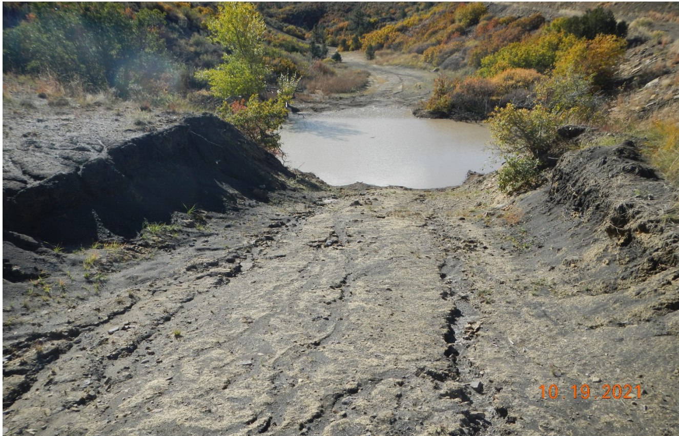
Photo 11. Facing south toward the road that was built to access the canyon bottom. There is erosion beginning to occur along this area which was not recontoured and reclaimed. Photo from previous inspection. See previous inspection details.
