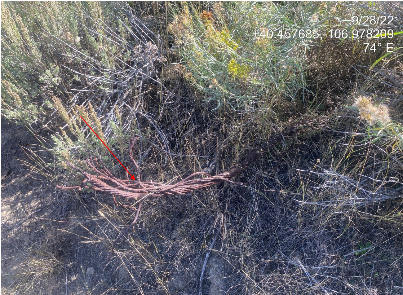
Photo 3. Photo taken directly adjacent to the pipe in Photo 2 shows a cable remaining in the fill slope at the west of the Location.
