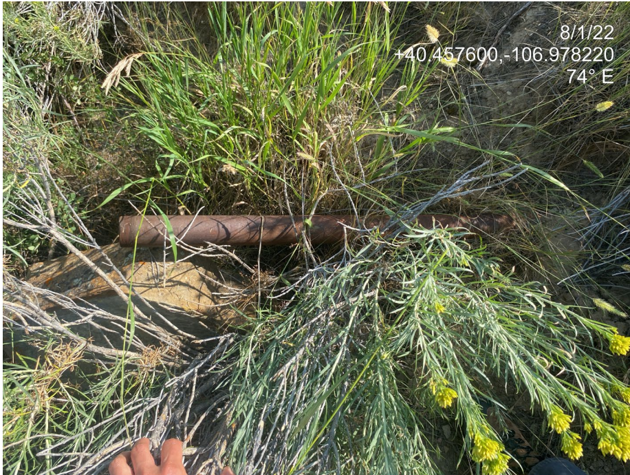
Photo 1. Photo from the 8/1/22 inspection showing a buried pipe coming out of the fill slope at the west of the Location, with approximate coordinates.
