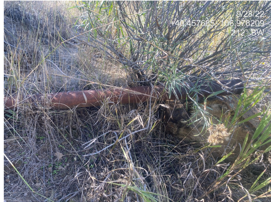
Photo 2. Photo from the 9/28/22 inspection showing the same buried pipe pictured in Photo 1 remaining in the fill slope at the west of the Location. Note approximate coordinates for location and removal of pipe.
