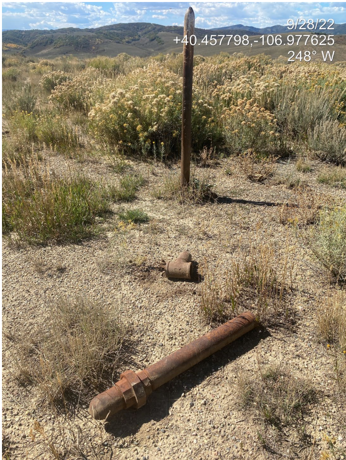
Photo 4. Photo taken from the well marker shows pipe debris found throughout the Location. Inspector piled debris for removal.
