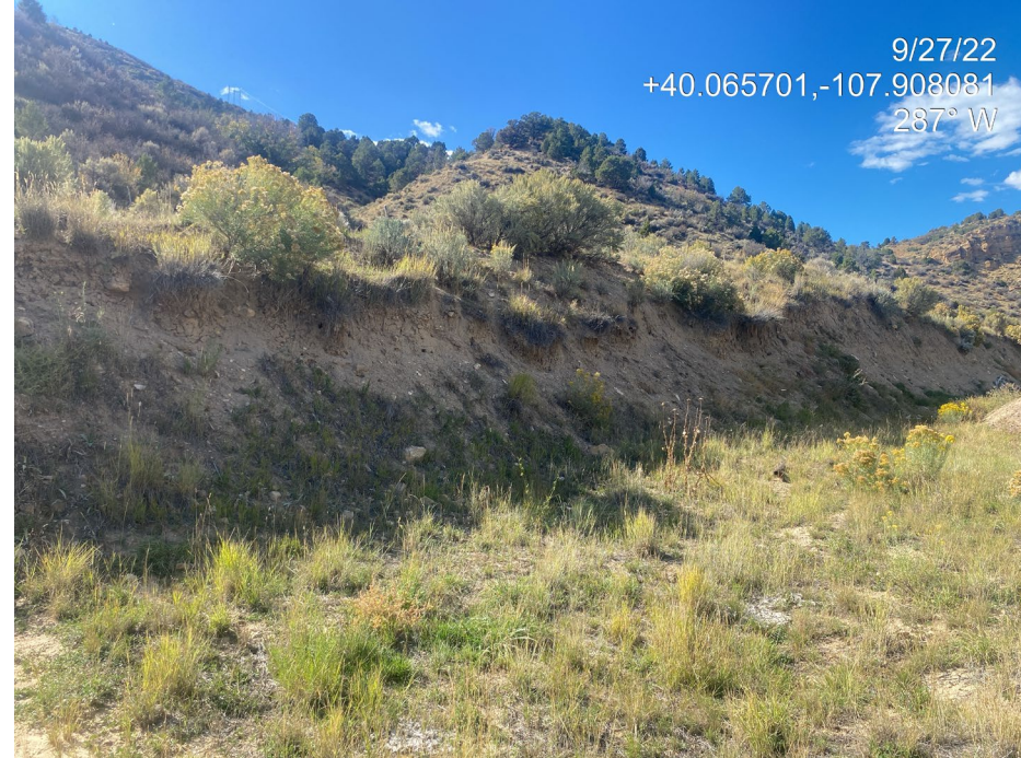
Photo 10. Photo taken from the west shows the eroded cut slope.
