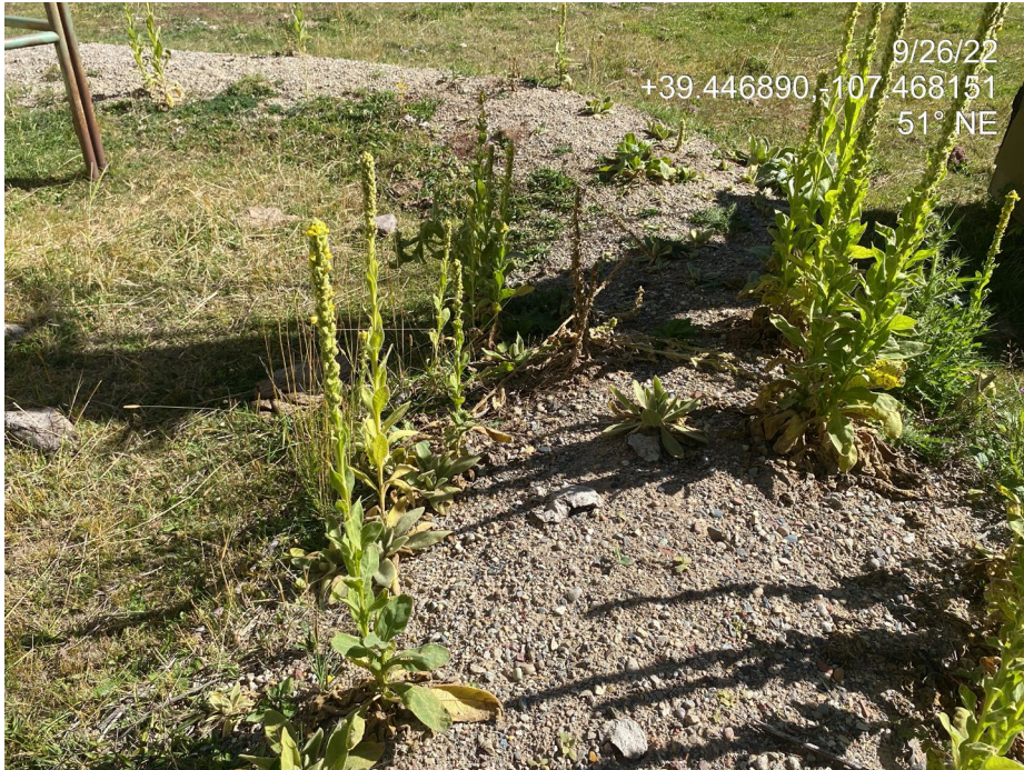
Photo 3. Photo taken from the south of the Location shows the tank secondary containment is not in proper functioning condition. The base of the secondary containment area is completely grown in with vegetation. The berm is eroded and compromised by vegetation growing on it. Species pictured include bull thistle (List B Noxious) and mullein (List C Noxious).
