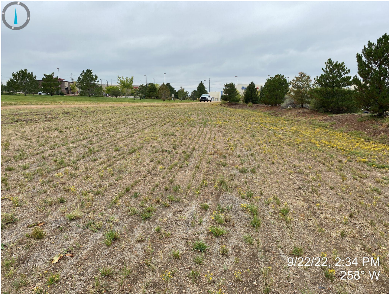
Photo 1. Taken from eastern portion, facing west. It appears operator has performed final reclamation activities with evidence of drill rows and desirable vegetation observed.
