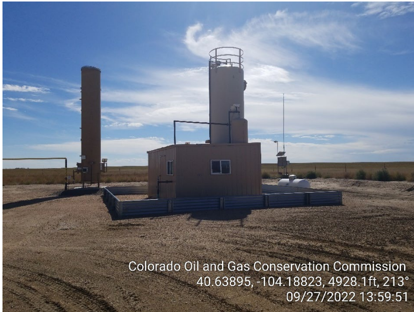
Photo 3 – ECD and Heater Treater
