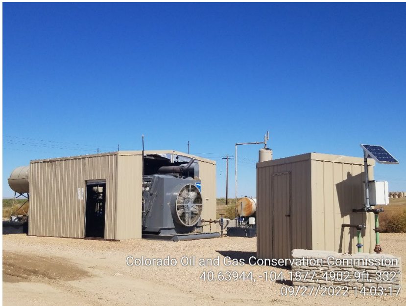
Photo 7 – Gas Lift Injection Meter Shed and Compressor
