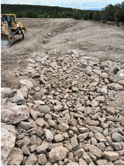
Angular rock and geotextile installed in northwest corner (facing southwest). BMPs also include rock check dams and diversion ditch.
