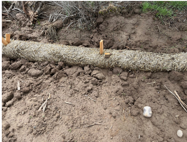
South side of location facing southeast, soil is no longer piled too high against wattles.
