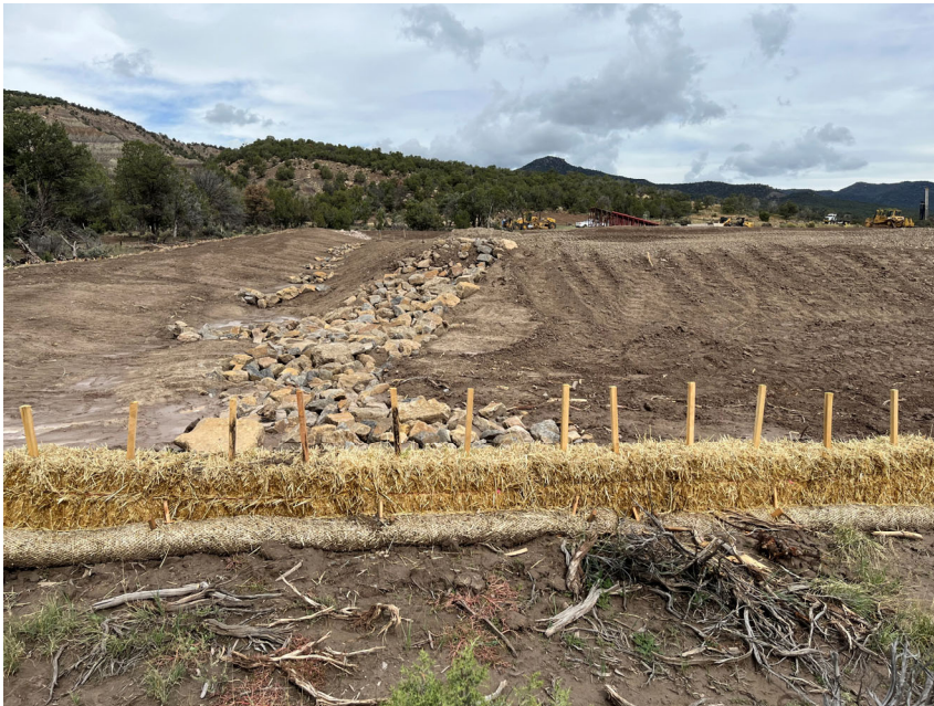
Southwest corner BMPs include diversion ditch with rock check dams, rock run down with geotextile material and angular rock, and straw bales.
