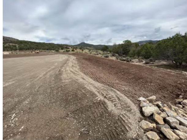
East side berm installed along pad edge to direct water to the rock rundown. Tracking perpendicular to slope.
