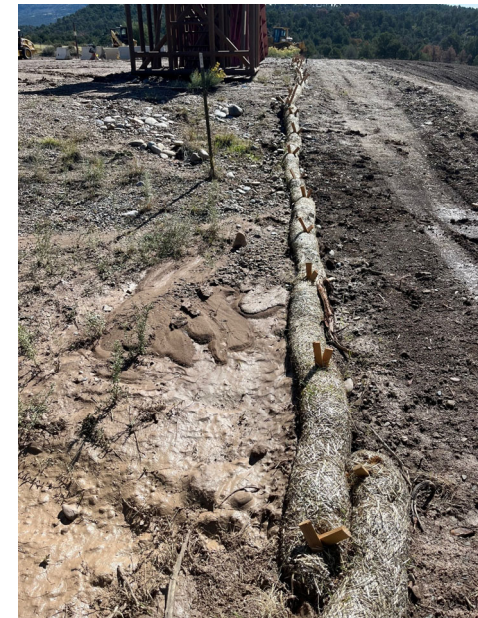
North side of pad, soil is no longer piled too high against wattles.
