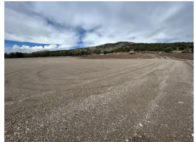
Pad surface grade finalized and aggregate applied.
