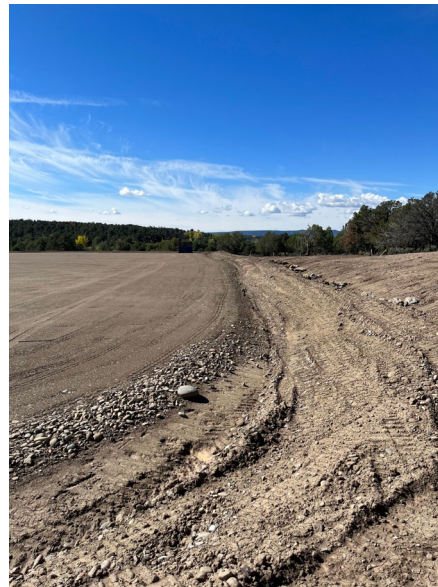
Pad surface grade finalized and aggregate applied.
