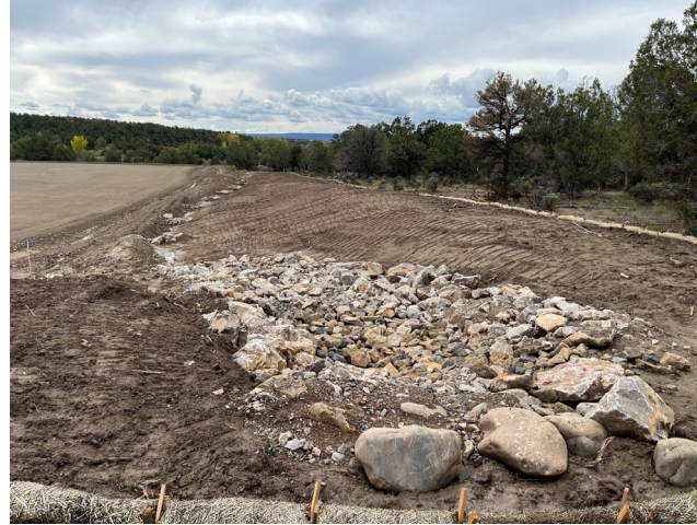
Angular rock and geotextile installed in northwest corner (facing southwest). BMPs also include rock check dams and diversion ditch.
