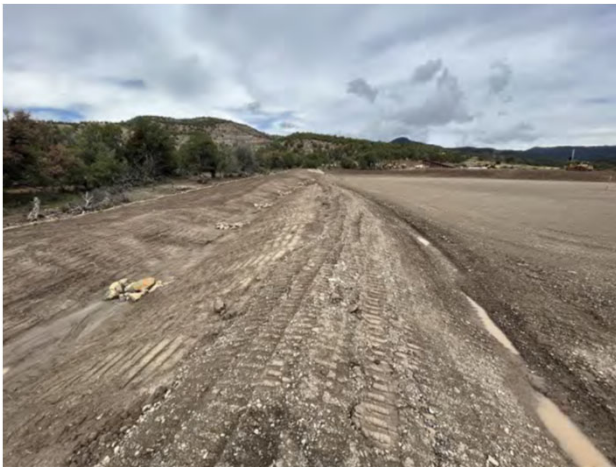
West side berm installed along pad edge to direct water to rock rundowns.
