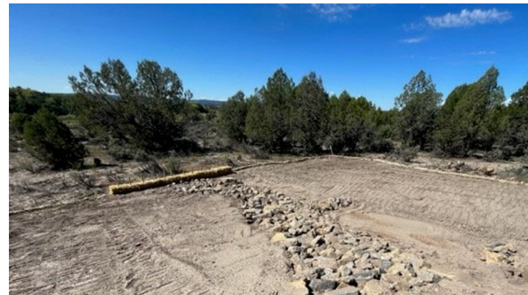
Southwest corner BMPs include diversion ditch with rock check dams, rock run down with geotextile material and angular rock, and straw bales.
