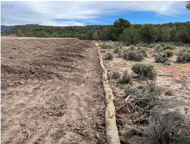
South side of location facing southeast, soil is no longer piled too high against wattles.
