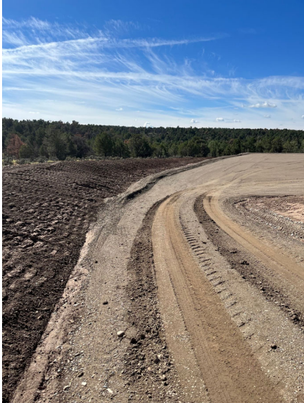
East side berm installed along pad edge to direct water to the rock rundown. Tracking perpendicular to slope.
