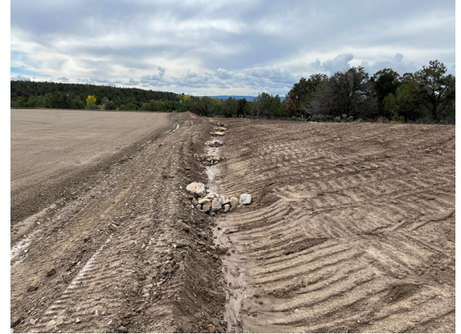
Angular rock and geotextile installed in northwest corner (facing southwest). BMPs also include rock check dams and diversion ditch.
