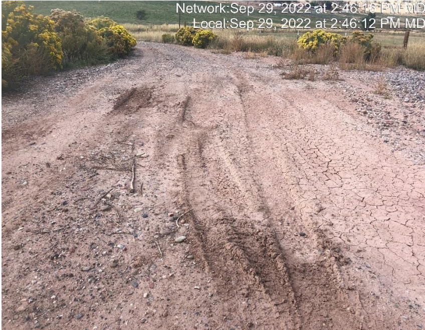
Photo #7880 Insufficient tracking BMP at entrance to location.
