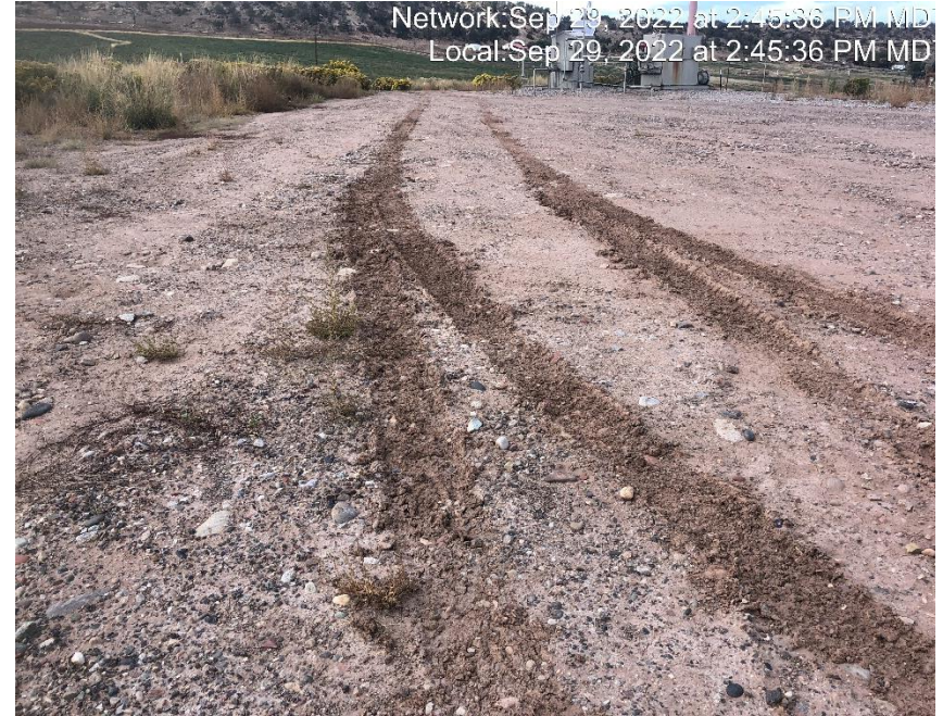
Photo #7879 Location lacks stabilization.
