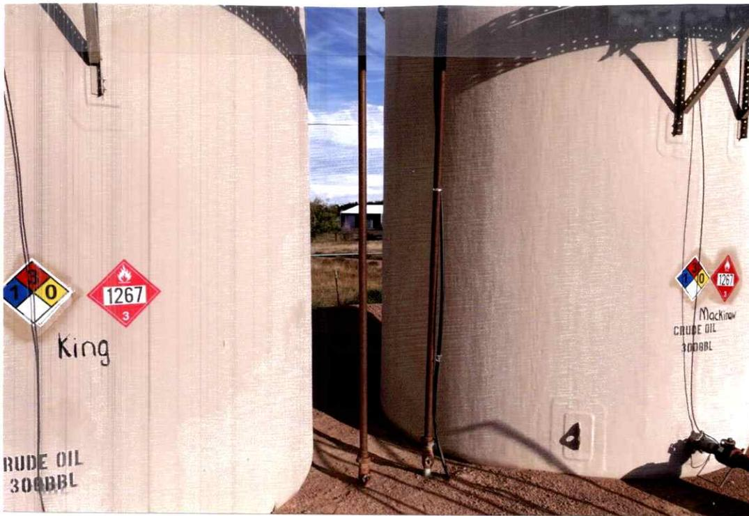
Tank labels (NFPA, Capacity, Contents). CA: Install sign to comply with Rule 605.h.
