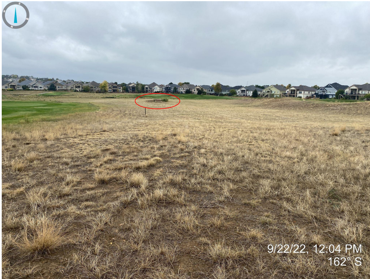
Photo 3. Taken north of location, facing south. Soil stockpile outlined in red. Photo illustrates former access road has been reclaimed with uniform vegetation cover and contoured/graded to reflect reference areas.
