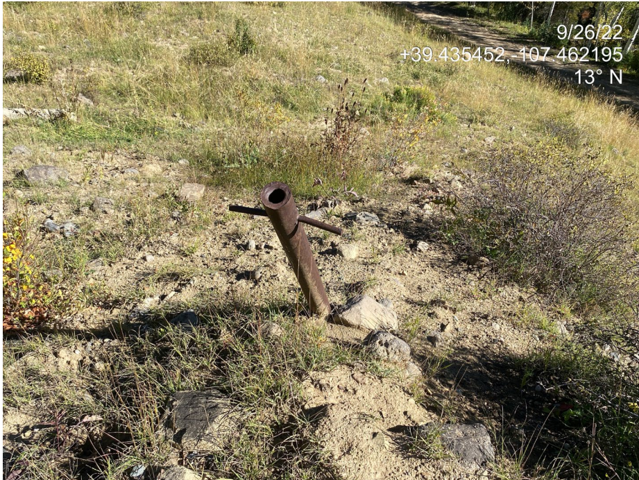
Photo 4. Photo taken from the north of the Location shows an example of unmarked anchor. All anchors on Location are unmarked.
