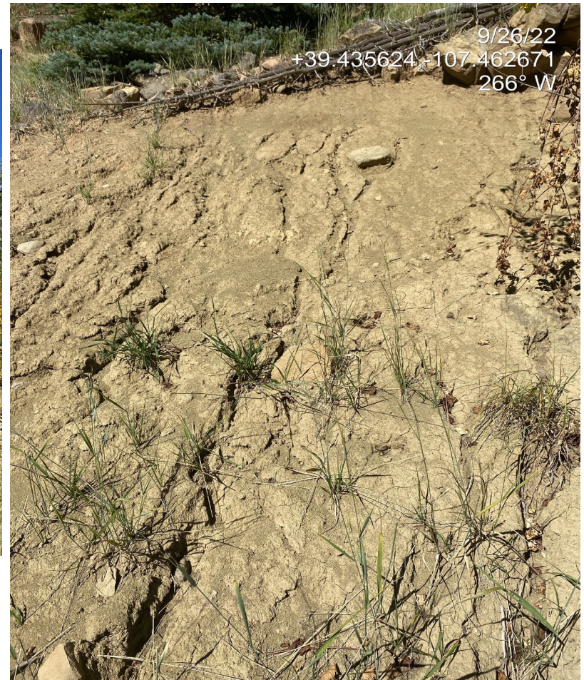
Photo 8. Photo taken from the north of the Location shows rill erosion occurring on the eroding cut slope.
