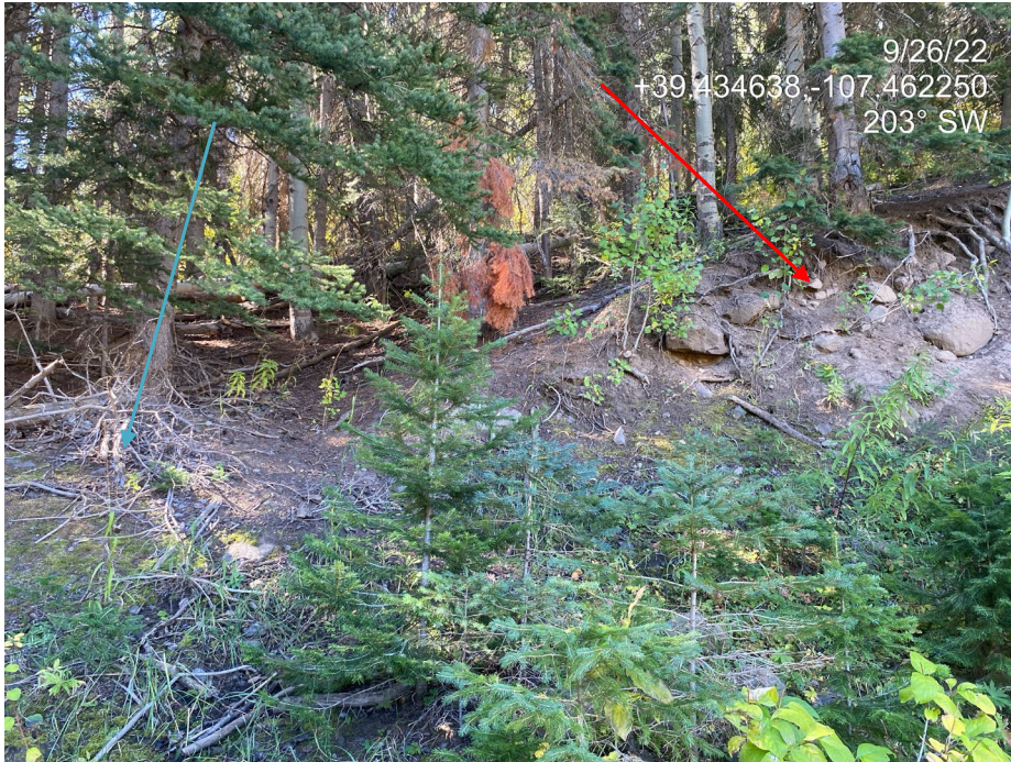
Photo 10. Photo taken from the south of the Location shows the slope/contour in the reference area (blue arrow) and the start of the Location cut slope (red arrow). The cut slope is eroding and undercutting into undisturbed areas above the cut exposing roots.
