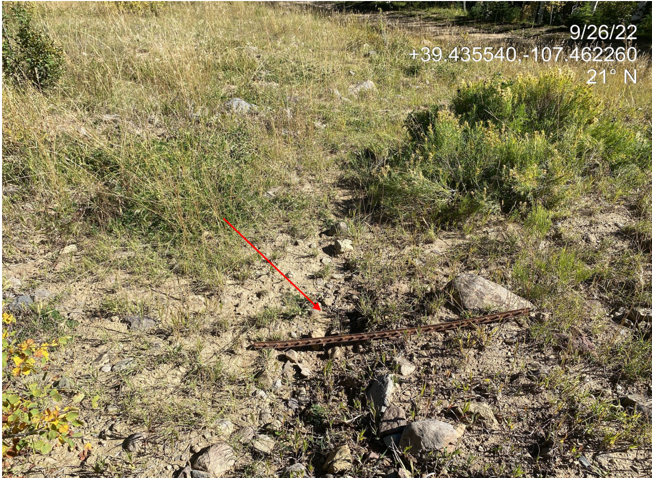
Photo 6. Photo taken from the north of the Location shows trash/debris. Photo also shows sediment deposition from the nearby cut slope and erosion occurring to the fill slope from stormwater flows coming off the cut.
