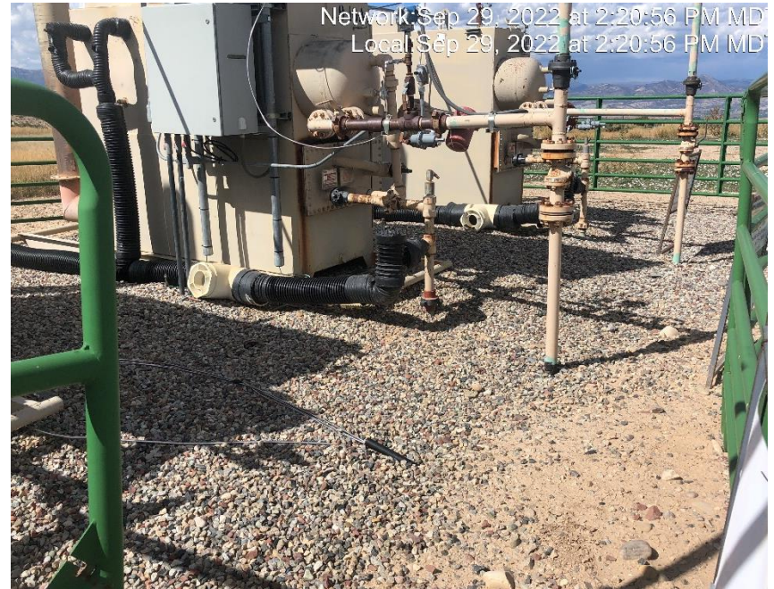
Photo #7861 Multiple places with heating insulation open ended and not capped.
