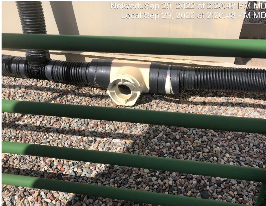
Photo #7860 Multiple places with heating insulation open ended and not capped.
