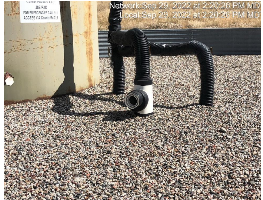
Photo #7859 Multiple places with heating insulation open ended and not capped.
