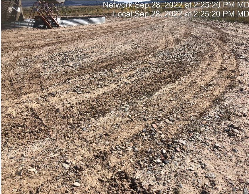
Photo #7847 Location lacks stabilization.
