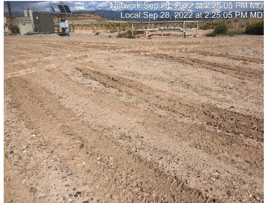
Photo #7844 Location lacks stabilization.
