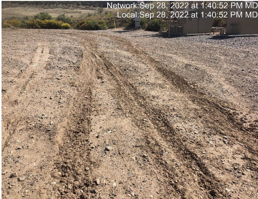
Photo #7833 Location lacks stabilization.
