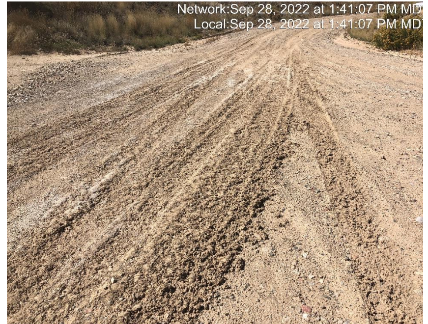
Photo #7835 Insufficient tracking BMP at entrance to location
