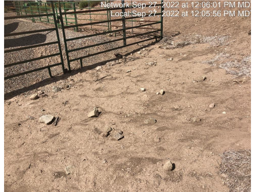
Photo #7802 Run on to location is not being controlled.
