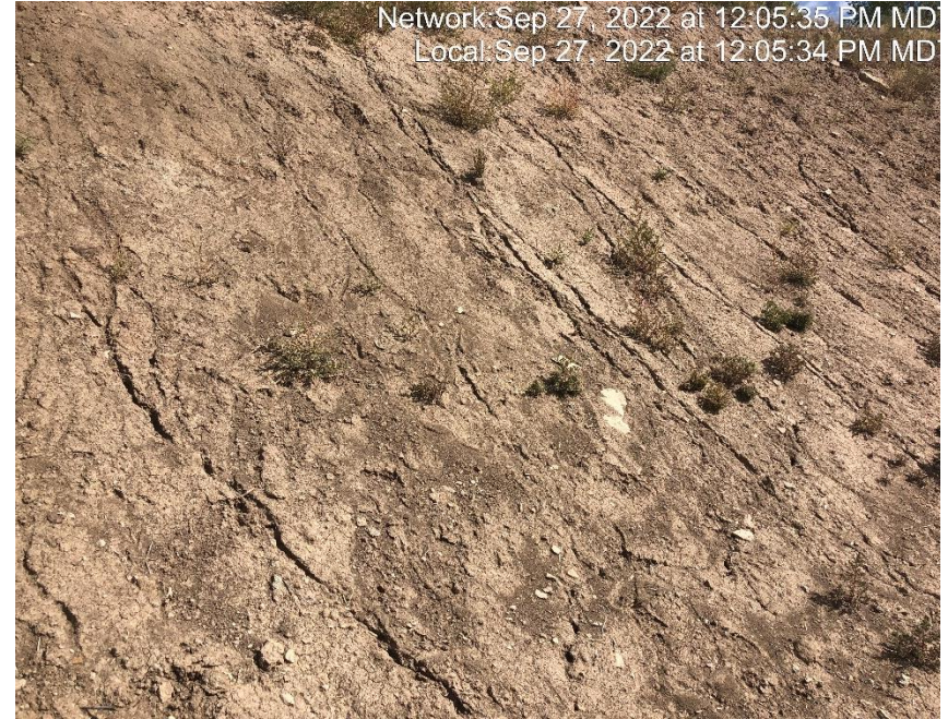
Photo #7800 Rill erosion occurring on cut slope.
