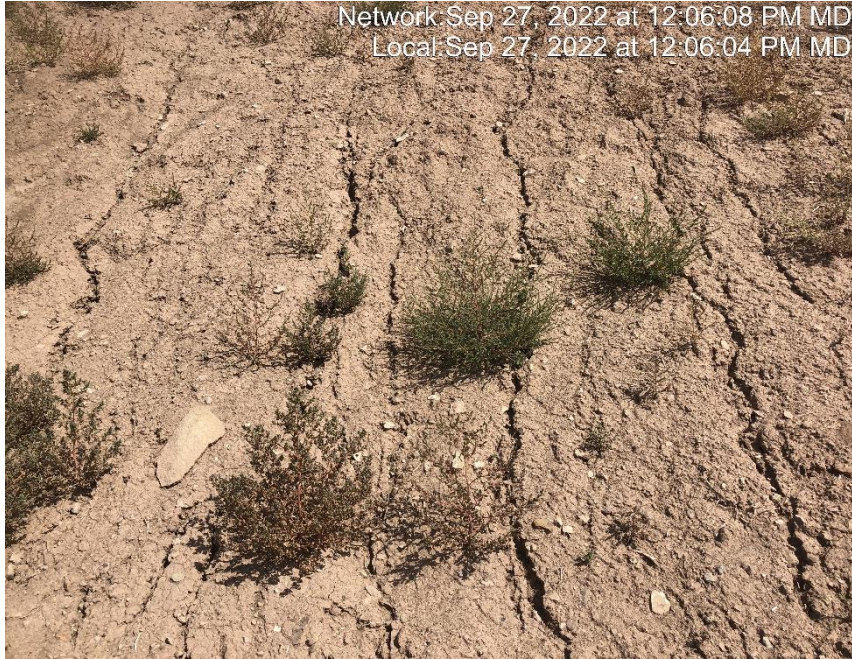
Photo #7803 Rill erosion occurring on cut slope.
