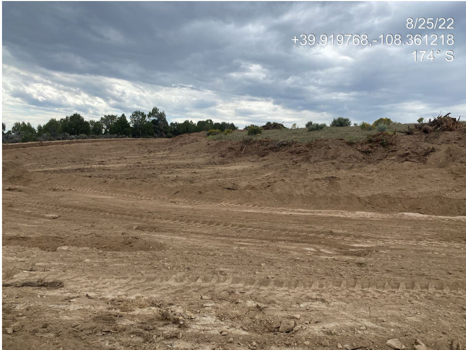
Photo 6. Photo taken from the northeast shows topsoil salvage taking place in the interim areas.
