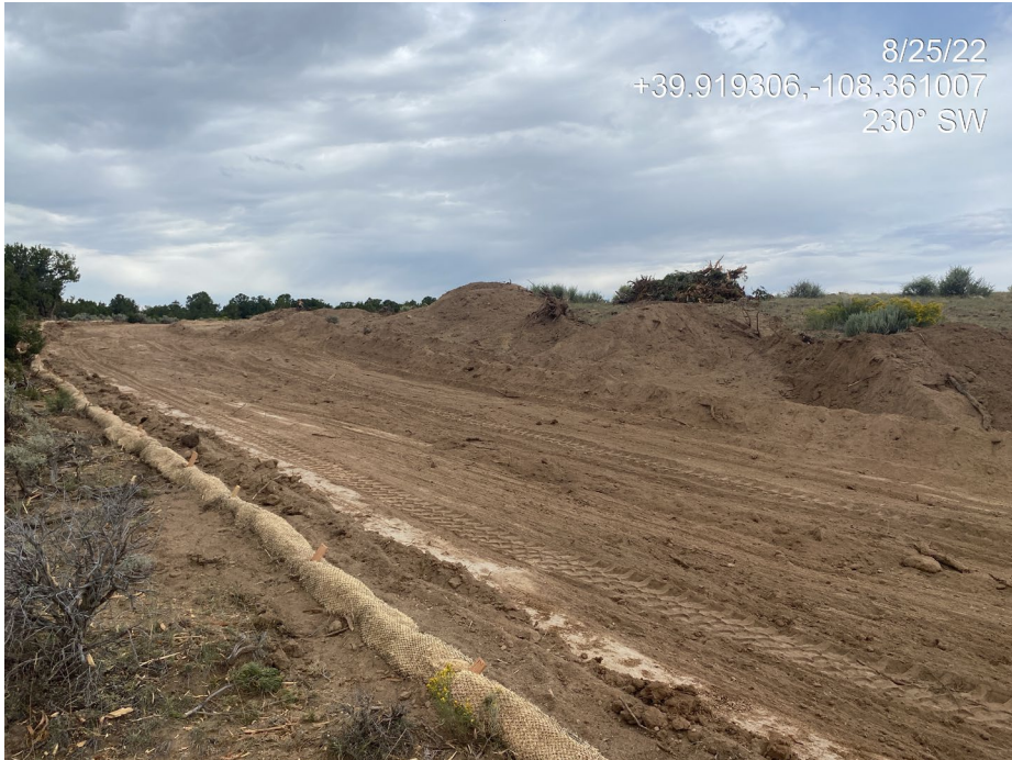
Photo 4. Photo taken from the southeast shows topsoil salvage taking place in the interim areas. Photo also shows a straw wattle installed around the perimeter of the Location.
