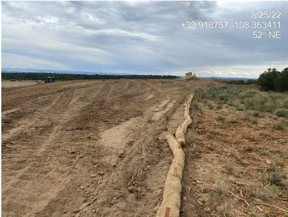
Photo 2. Photo taken from the southeast shows topsoil salvage taking place in the interim areas. Photo also shows a straw wattle installed around the perimeter of the Location.
