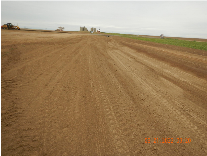
Photo 3. Photo taken from the eastern location, facing North. Photo illustrates a ditch and berm BMP installed around the perimeter of location which is directed to a retention area.
