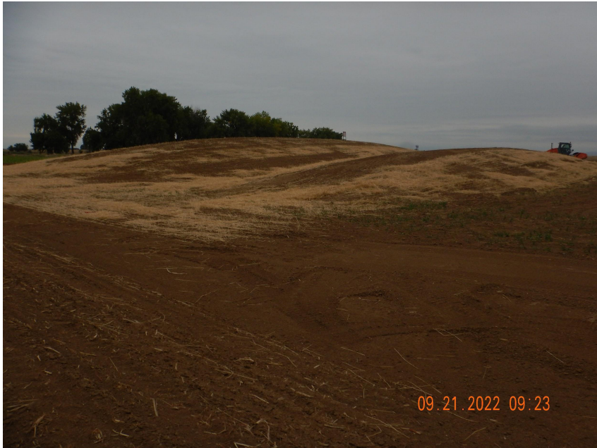
Photo 5. Photo taken from the southeastern location, facing Southwest. Photo illustrates the topsoil stockpile has been seeded and straw crimped with mulch. However, the straw crimped mulch has blown off most of the stockpile; therefore, CDPHE is requiring a corrective action.
