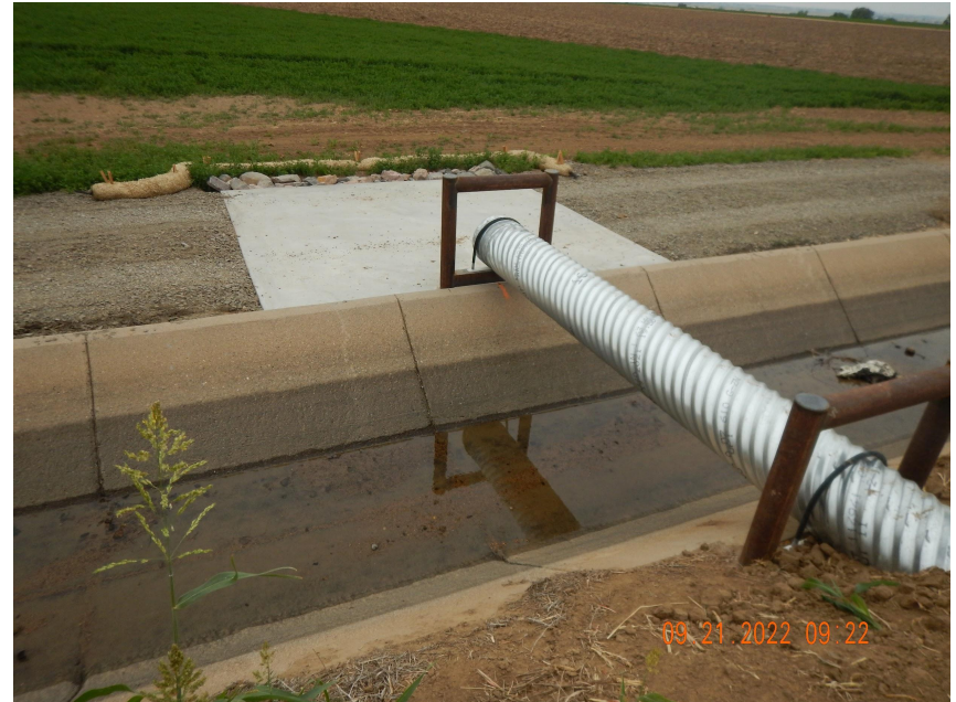
Photo 4. Photo taken from the eastern location, facing East. Photo illustrates the overflow outlet. Stormwater discharge would not be accepted into the irrigation ditch.
