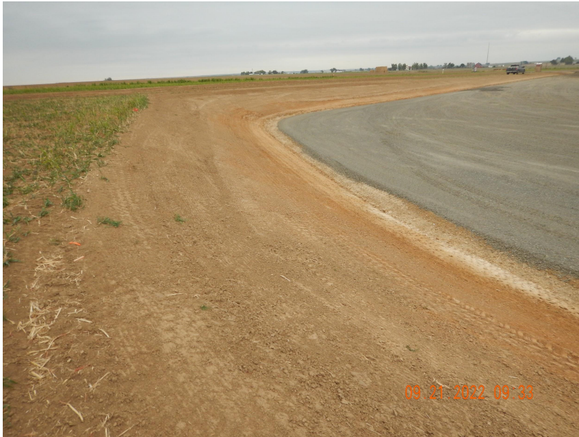
Photo 7. Photo taken from the northwestern location, facing North. Photo illustrates the cut slope may need further stabilization to ensure long-term stabilization.
