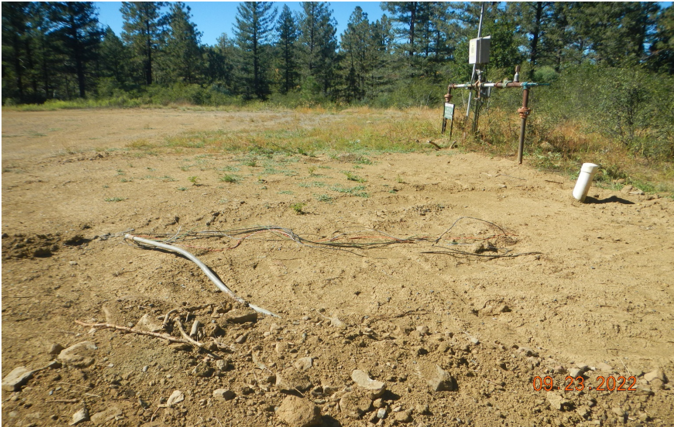
Photo 4. Facing northwest toward the wellsite. There are exposed electric lines on the surface. The lines need to be removed or repaired and protected. This area of disturbance needs to be seeded and stabilized.
