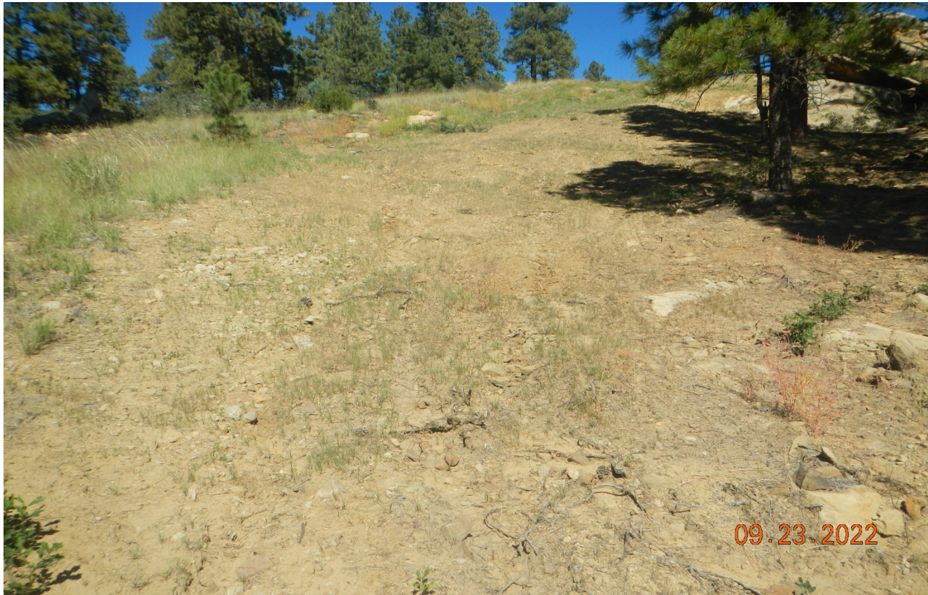
Photo 1. Facing northwest at the disturbance along the gathering pipeline at Lat/Long:37.05440,-104.76614. This area has been reseeded however, soils are not stabilized and there is now erosion occurring. Previous corrective action not completed.
