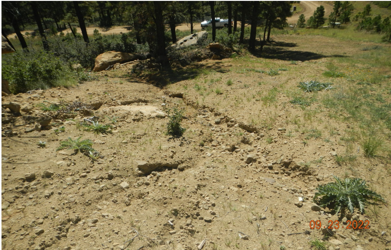
Photo 4. View of some of the erosion occurring. Additional BMP's are needed to prevent erosion. Previous corrective action not completed.
