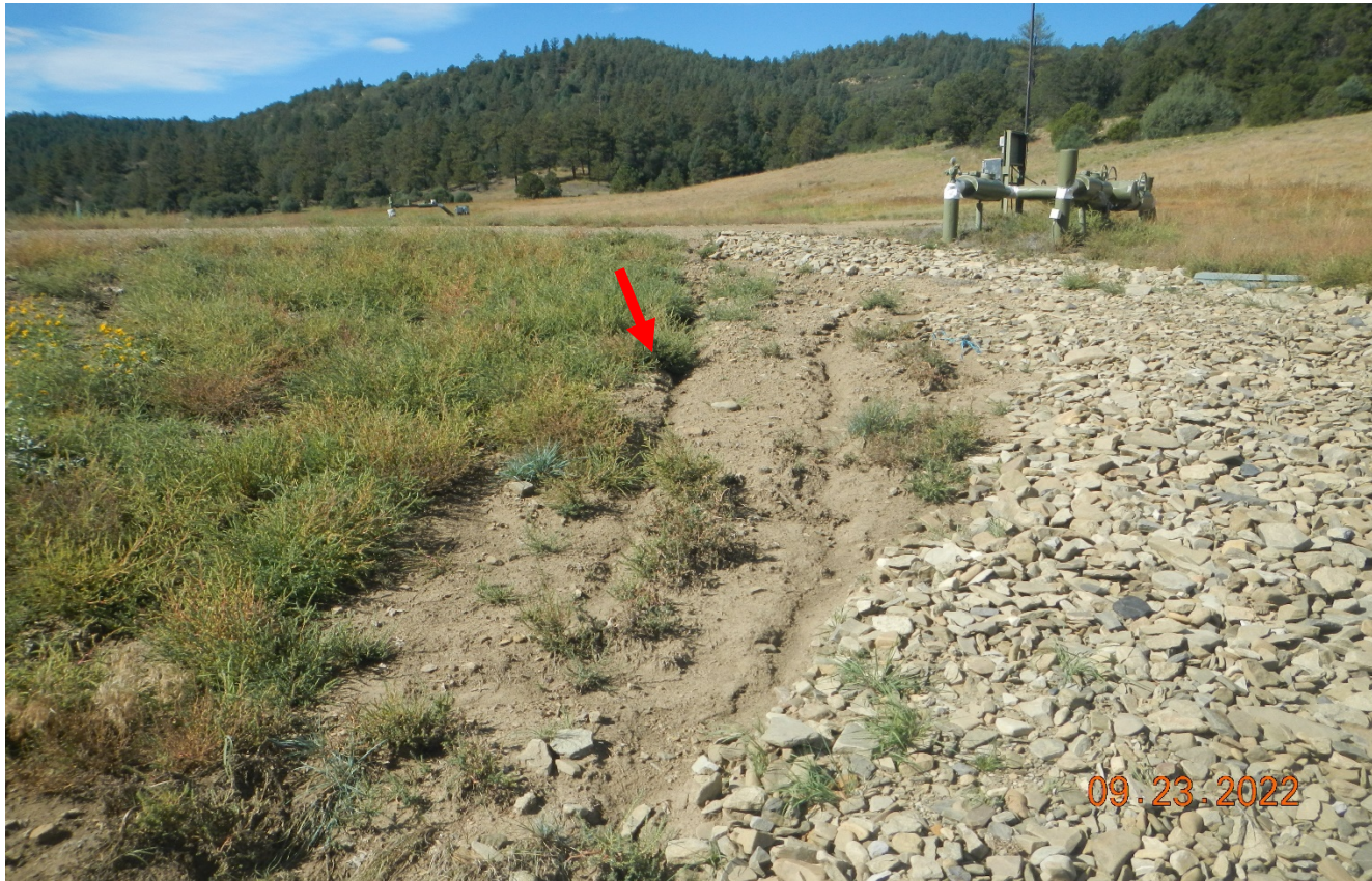
Photo 5. Facing southwest. There was rock rip/rap placed in this area where erosion had occurred. Stormwater is now going outside of the rip/rap area causing erosion at red arrow. Additional BMP's need to be installed in this area.
