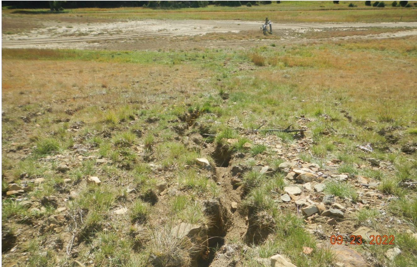
Photo 6. Facing east toward the location at the upper cut slope area. Stormwater run-on is causing erosion and is not properly diverted by the perimeter ditch. This area needs to be repaired and stabilized. Previous corrective action is not completed.
