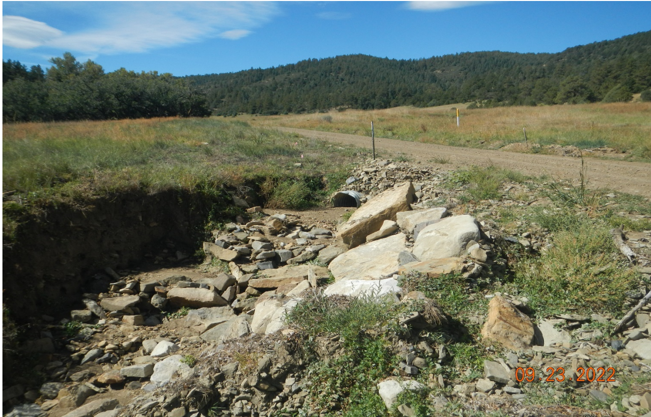
Photo 1. The culvert outlet has eroded and needs to be repaired. Previous corrective action was not completed.
