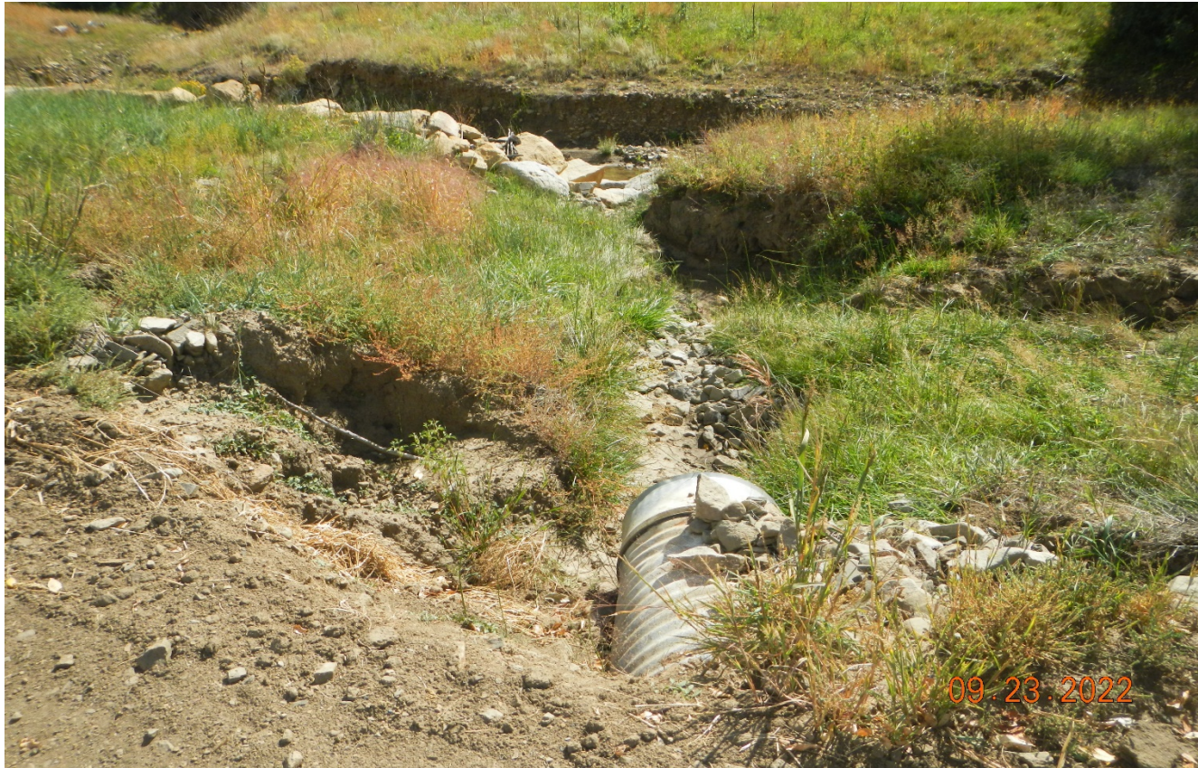
Photo 3. The next culvert along the road is also eroded at the culvert outlet with no outlet protection.
