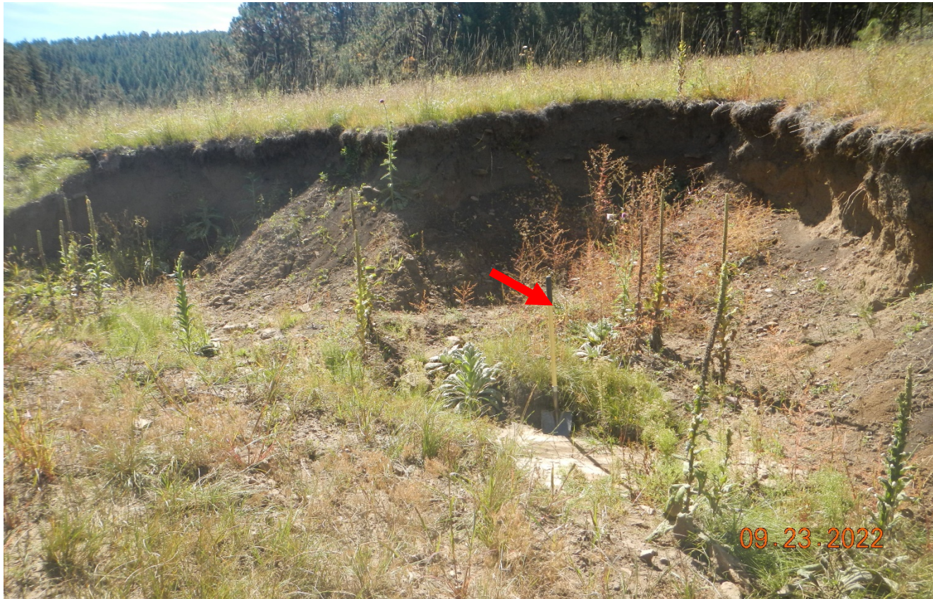
Photo 5. The side of the road is eroded and not stabilized. Erosion head cutting is continuing to occur further back. This area needs to be repaired and stabilized. Previous corrective action not completed. Red arrow points to 4.5 ft. shovel. Lat/Long:36.99952,-104.83425. There are also noxious shown in the photo.
