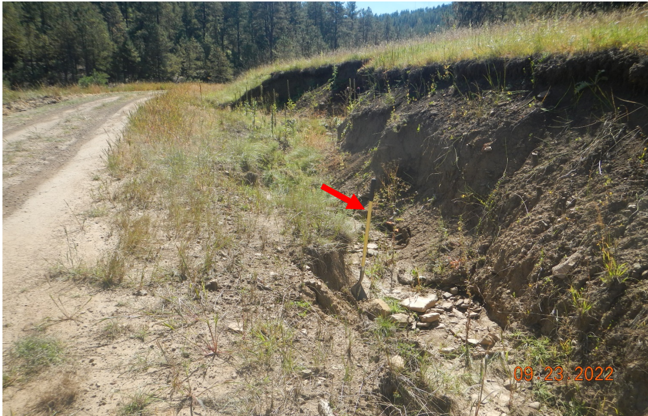
Photo 4. The side of the road is eroded and not stabilized. This area needs to be repaired and stabilized. Previous corrective action not completed. Red arrow points to 4.5 ft. shovel. Lat/Long:36.99952,-104.83425.
