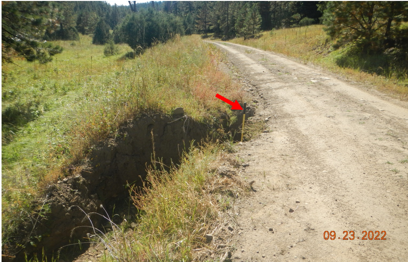
Photo 3. There is an erosion gully along the road that needs to be repaired and stabilized. Previous corrective action was not completed. Red arrow points to 4.5 ft. shovel.
