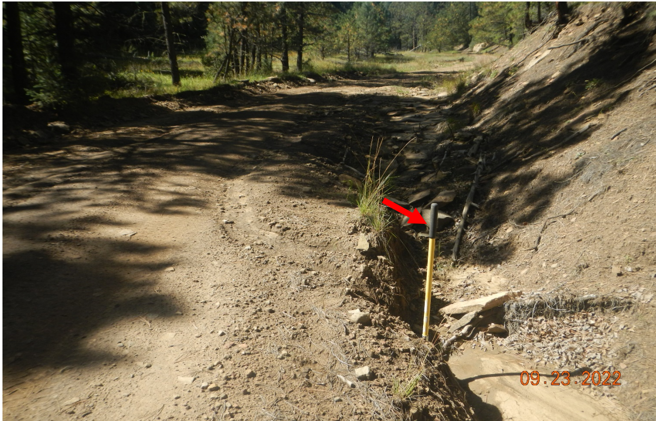
Photo 6. Further along the road near the Colorado line. The roadside and road is eroded and needs to be repaired and stabilized. Red arrow points to 4.5 ft. shovel.
