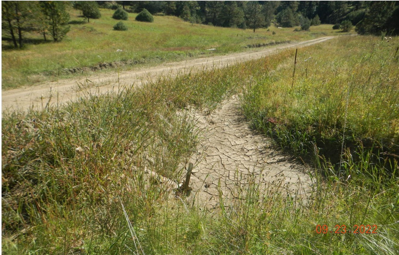
Photo 1. This culvert inlet was cleaned out however, the culvert is full of sediment. Previous corrective action was not completed. Lat/Long:37.00581,-104.83861.
