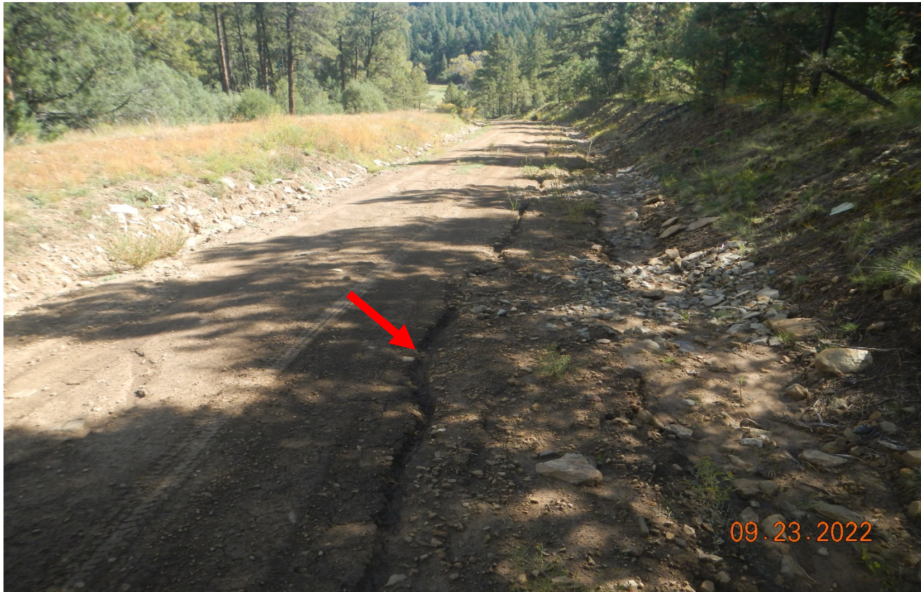
Photo 6. Further along the road facing back east. There is stormwater erosion occurring down the road which will continue to worsen since the previous inspection.
