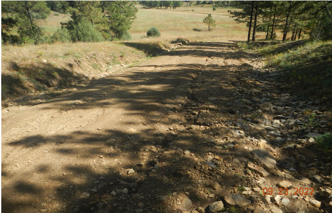
Photo 4. There are signs stormwater is flowing down the road causing erosion. This area has been a problem before. Stormwater is not being properly diverted off the road.
