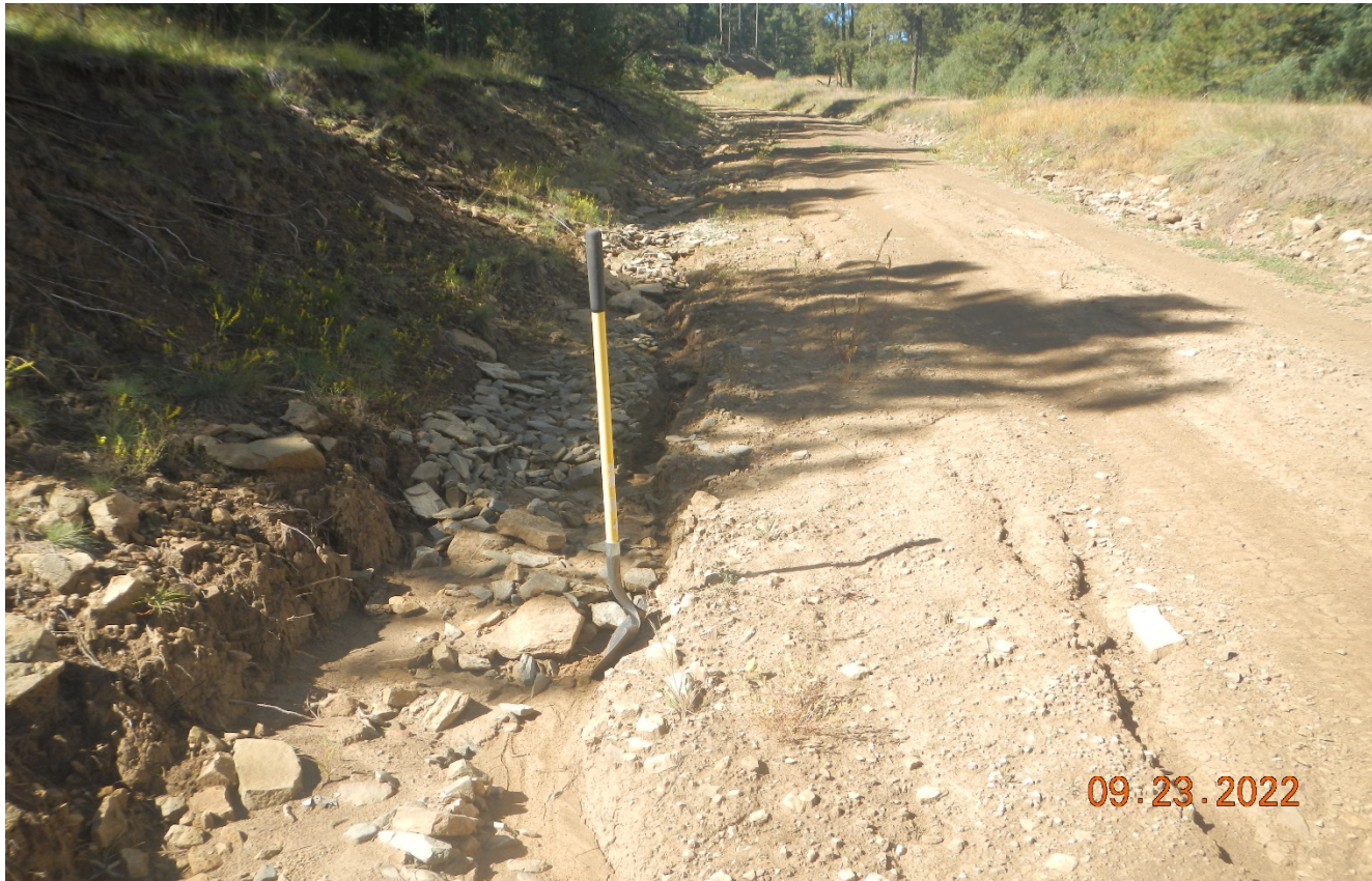
Photo 5. Facing west along the access road. Some of the rock check dams previously installed have washed out. Larger rock was likely needed. A 4.5 ft. shovel shows scale of erosion.
