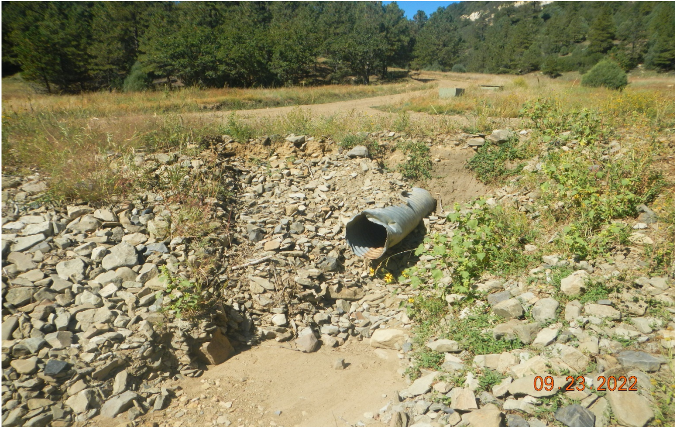
Photo 2. Facing west toward near the access road ascending the hillside. The culvert outlet has been washed out from recent storm event. It appears a larger culvert is needed along with larger rock rip/rap outlet protection.
