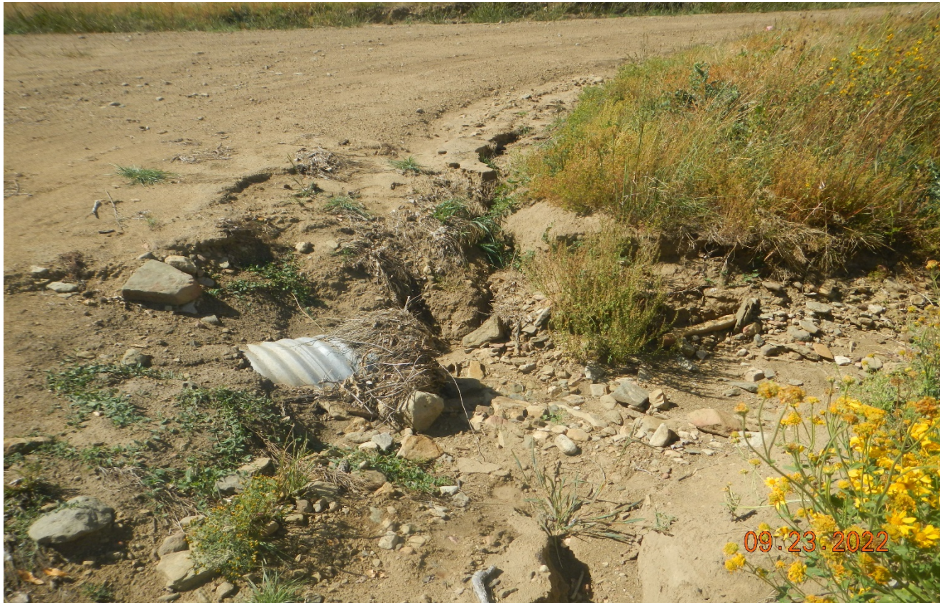
Photo 3. The culvert inlet is filled in with sediment and debris. It appears a larger culvert is needed at this area to handle stormwater coming off the road and drainage.
