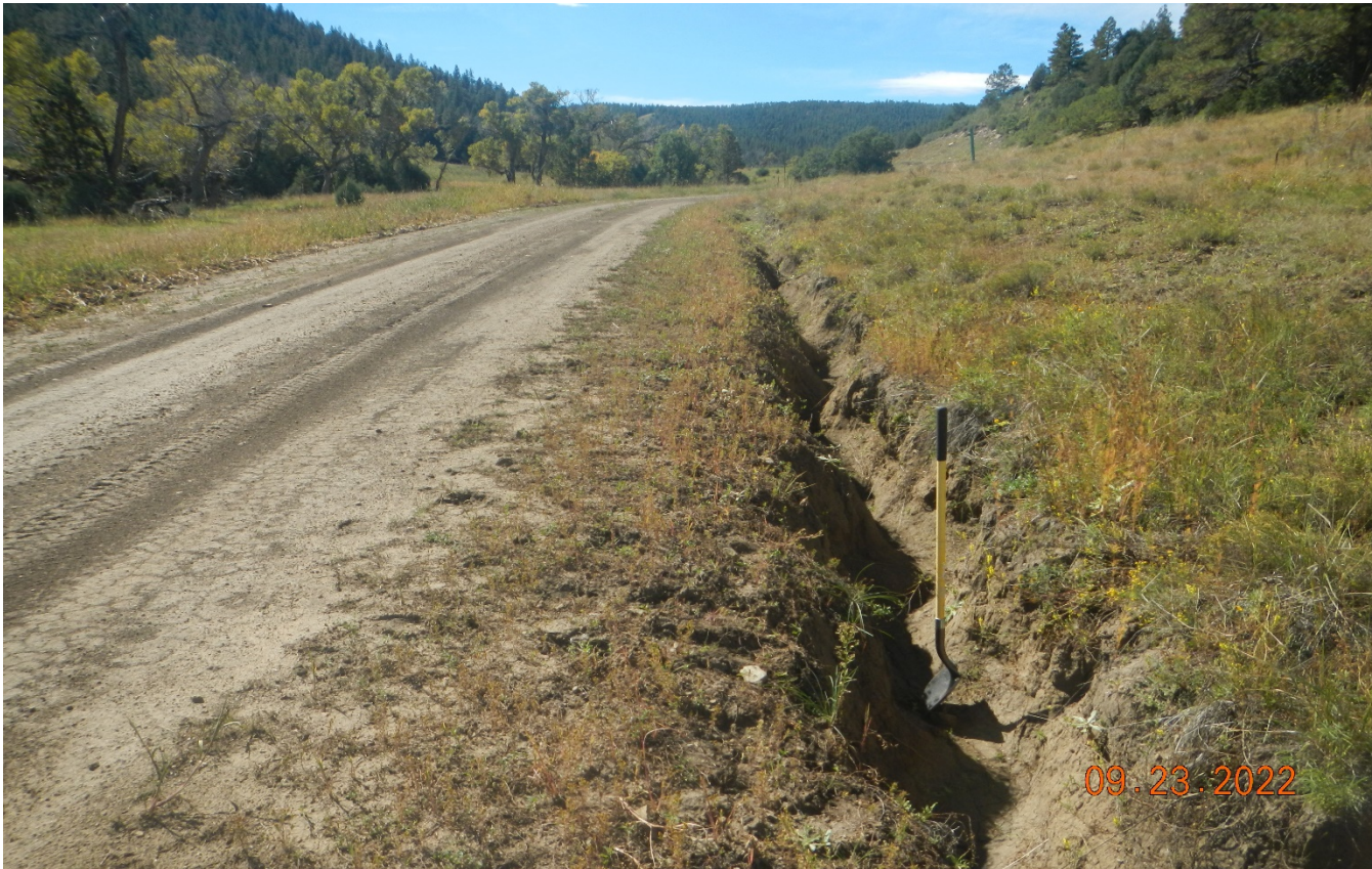
Photo 1. Facing south along the main road. There is erosion occurring along the road side. BMP's need to be installed to prevent erosion.
