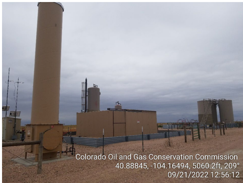
Photo 1 – Heater Treater and ECD
