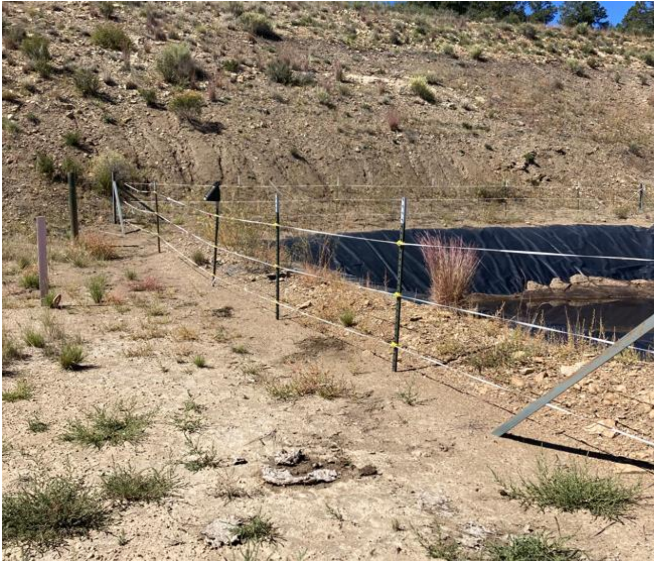
PHOTO 1: THE FENCING AROUND THE LINED PIT HAS BEEN REPAIRED TO COMPLY WITH THE REQUIREMENTS PER THE 1002A RULES.
